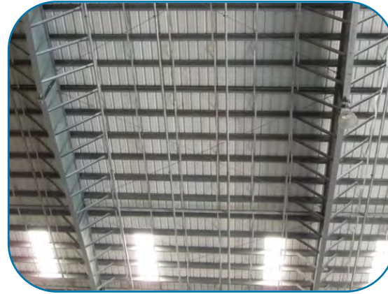
Reinforced Dry Stacks
