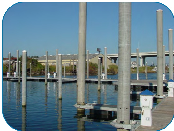
Pilings – 70 ft & 16 in diameter
