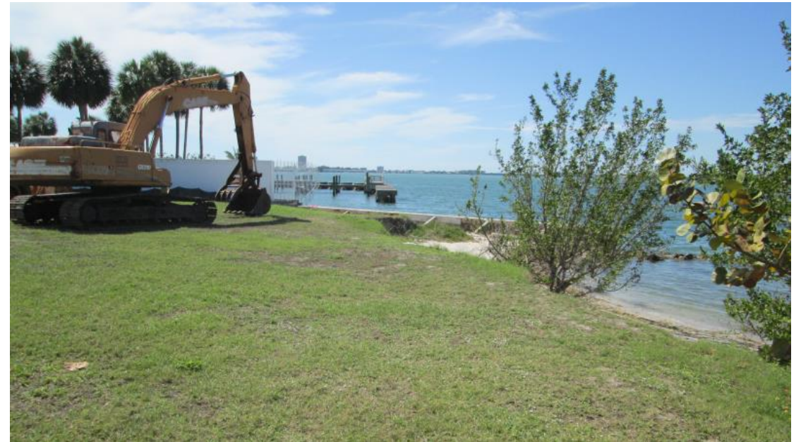
Removal of the existing seawall
