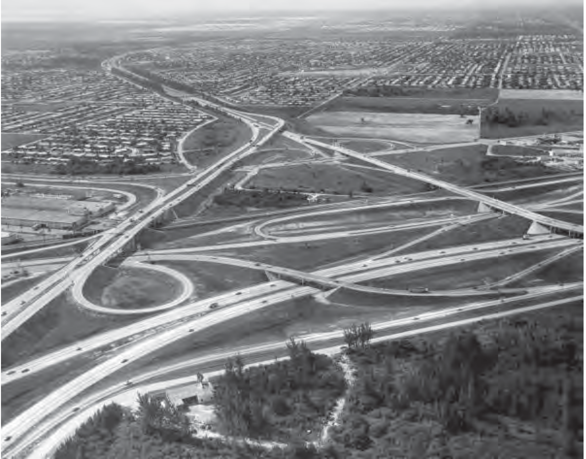
The intersection of Interstate-95 and the Florida Turnpike in North Miami in 1967. Today more than twice as many people make their homes in the Miami-Dade County area . Florida Photographic Archives.
