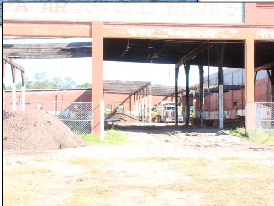
Soil removal inside trolley barn
