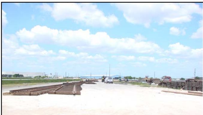
Relocation of railroad line through Winner Metals site
