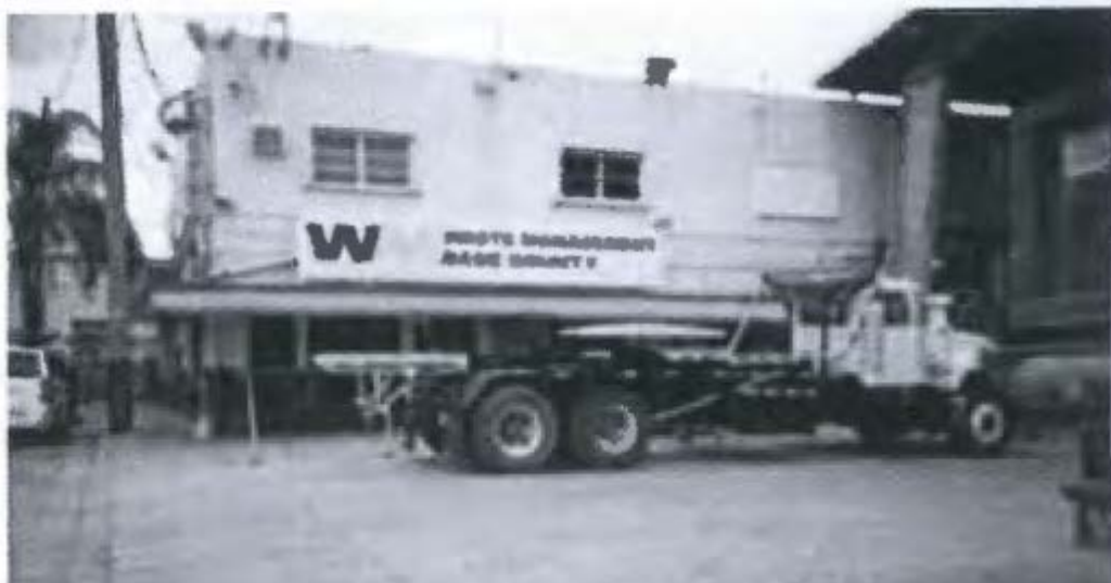
Former Waste Management Facility
