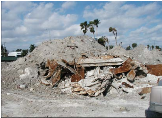
Solid Waste Removal
