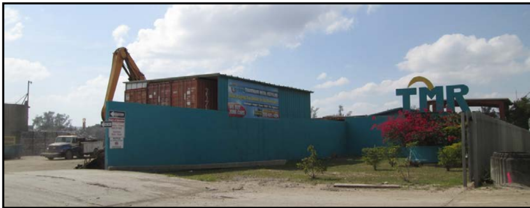
Trademark Metals Recycling Facility (2014)
