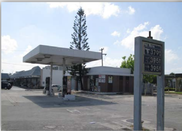
Out of service gas station (2014)
