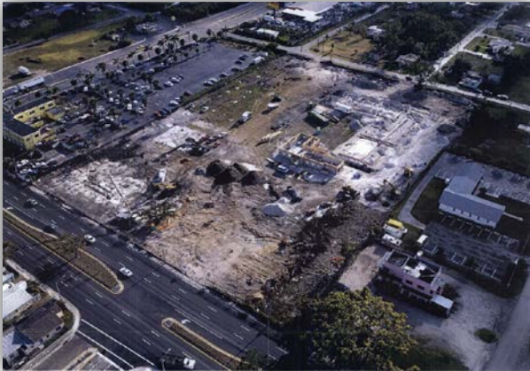
Prior to site construction (April 13, 2006)
