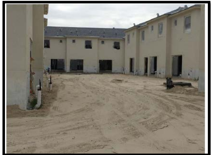
New construction - December 2016
