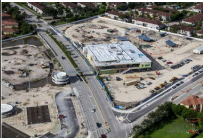
Site development - September 2016
