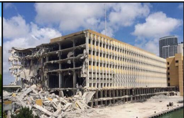
Demolition of Miami Herald Building (2014)
