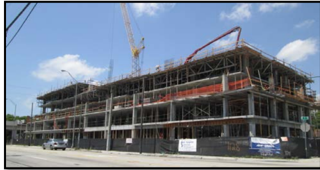
Site construction (May 2014)
