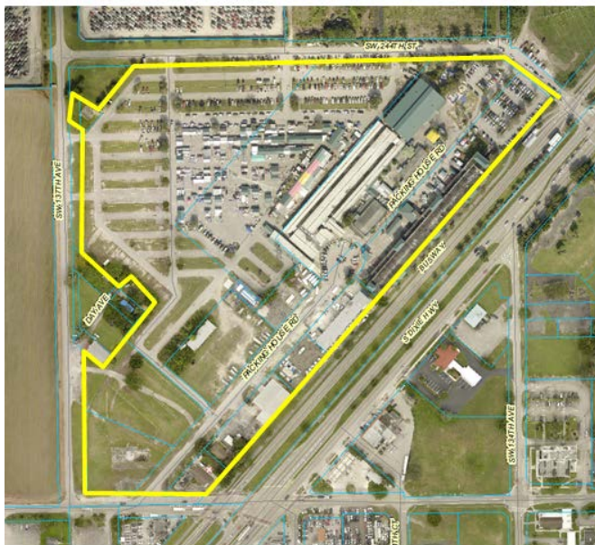
Redland Market Village Site
