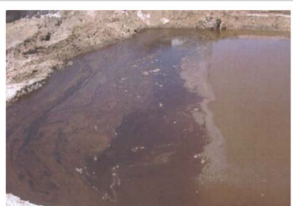
Free floating product in excavation
