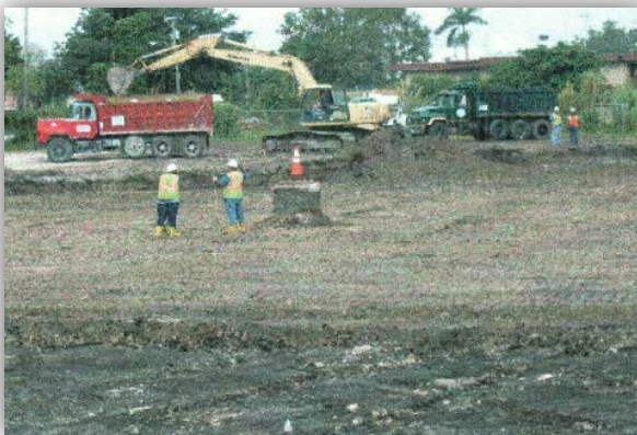
Soil and ash removal
