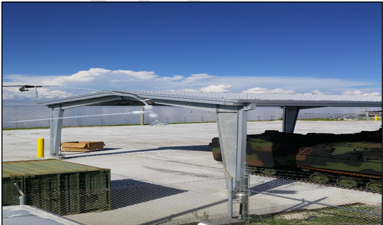
Figure 2.8 Northwest from the Site
