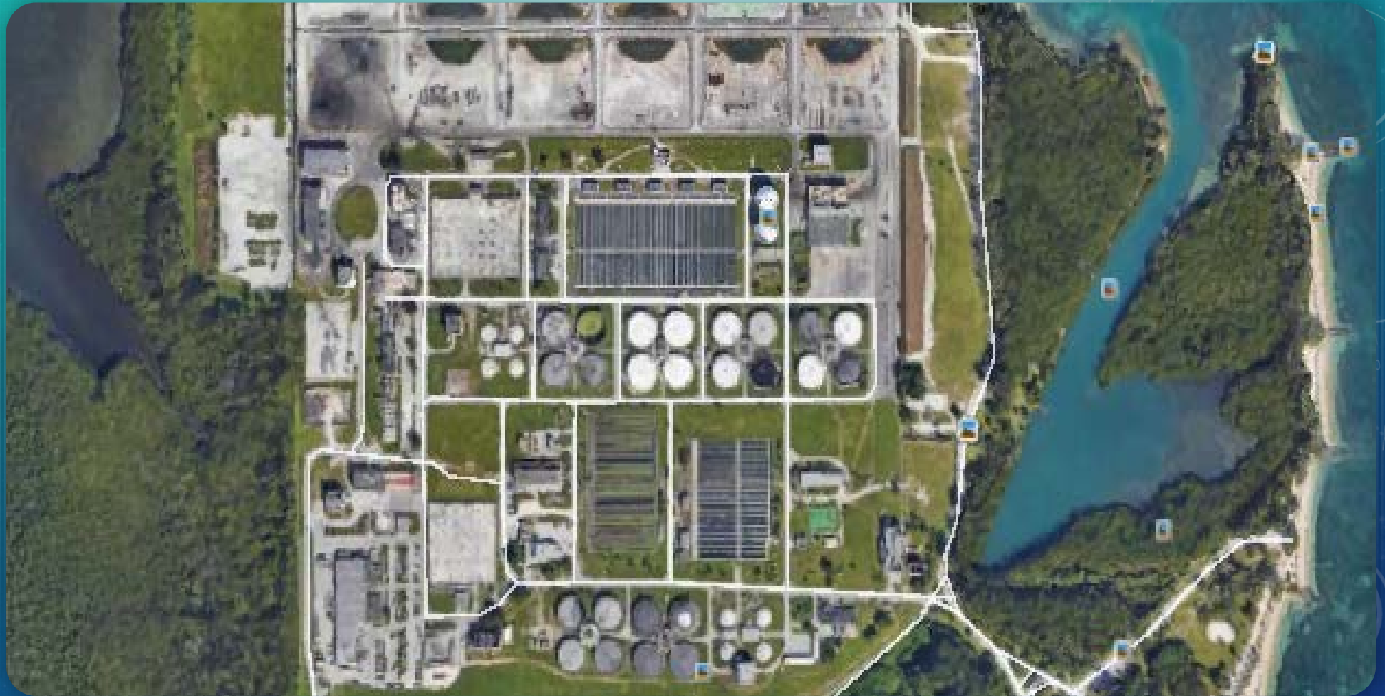
Wastewater Plant on Virginia Key, Miami
