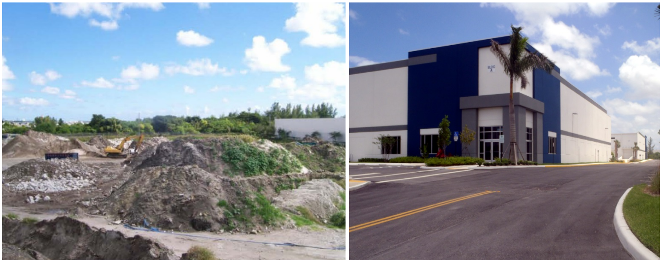
Above: The Dania Motocross Site in 2010 (left) and after rehabilitation and redevelopment in 2015 (right)
