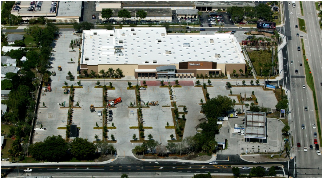
The Wal-Mart Neighborhood Market in Pompano Beach
