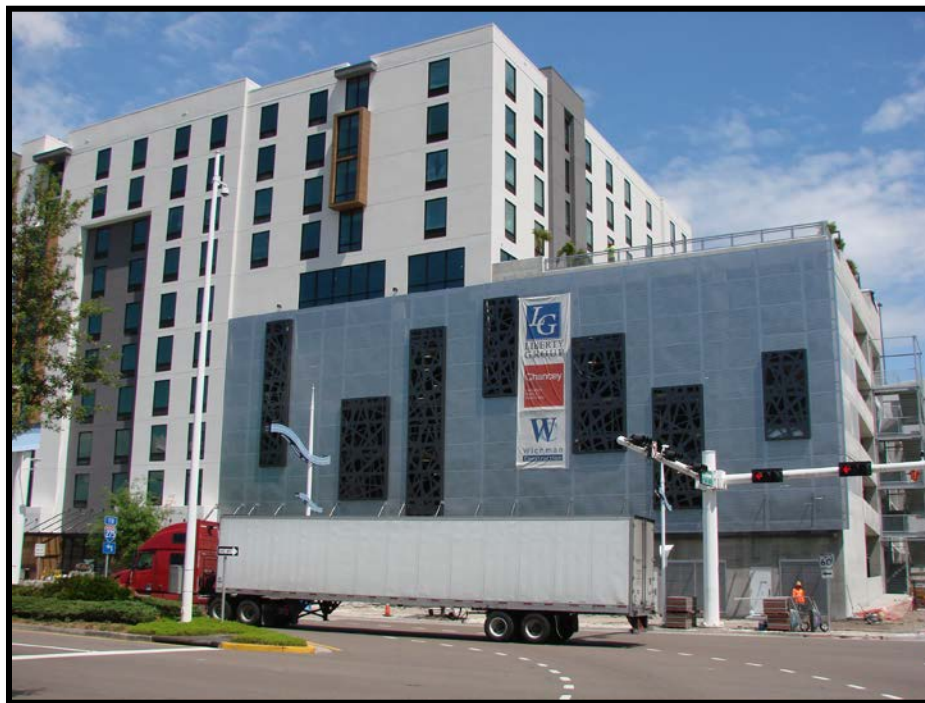
Liberty Tampa site at construction end, March 2019
