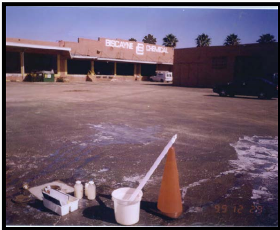
Exterior of site (1999)
