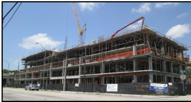
Site construction - May 2014
