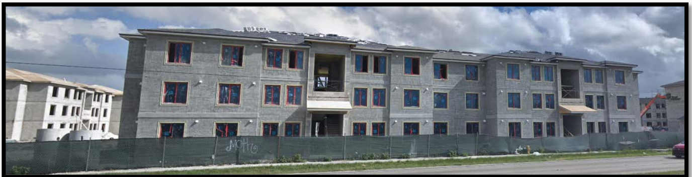
Construction on-going (May 2019)
