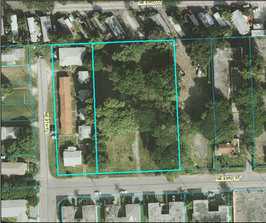
Site prior to demolition
