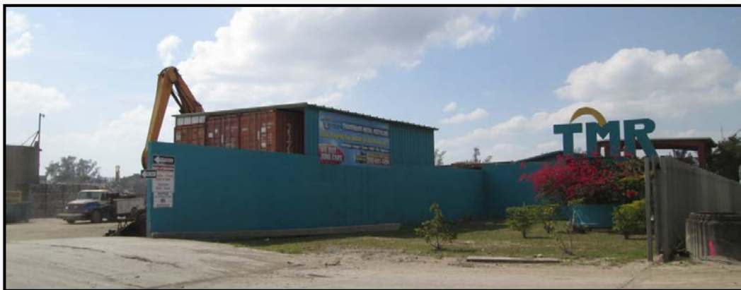
Trademark Metals Recycling Facility
