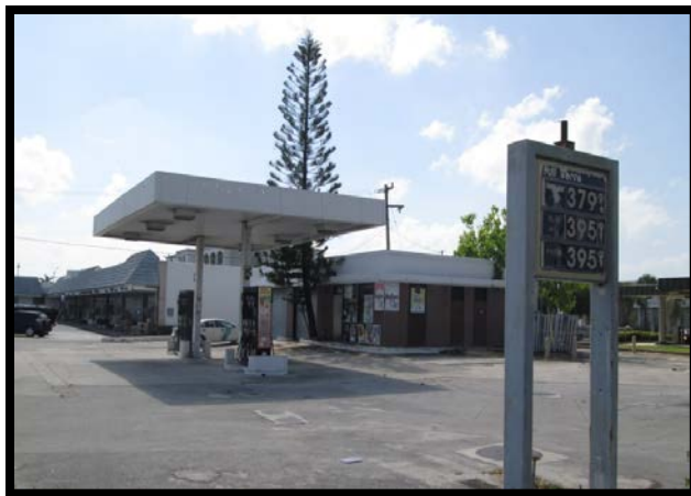
Out of service gas station (2014)
