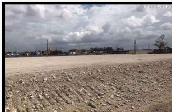
Site with 2-foot clean fill cap (2019)
