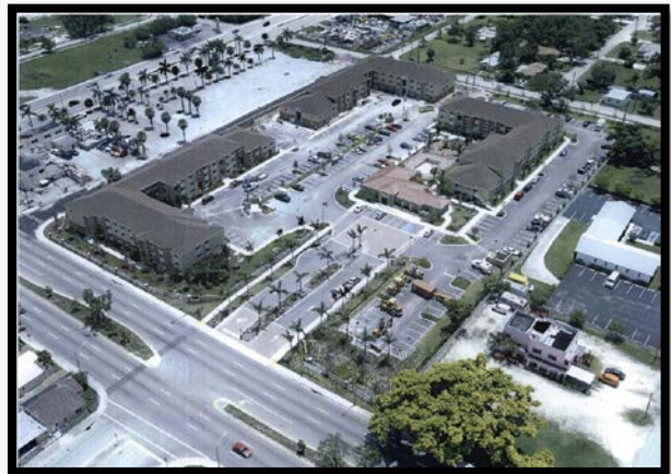
The Corinthian completed (June 8, 2007)
