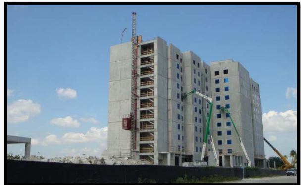
Adjacent building construction (2015)
