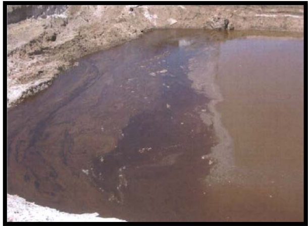
Free floating product in excavation
