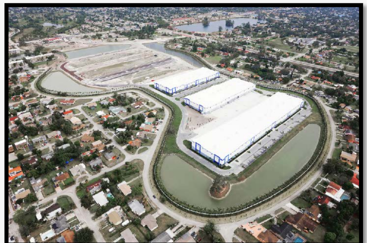
Site development in process - January 2019
