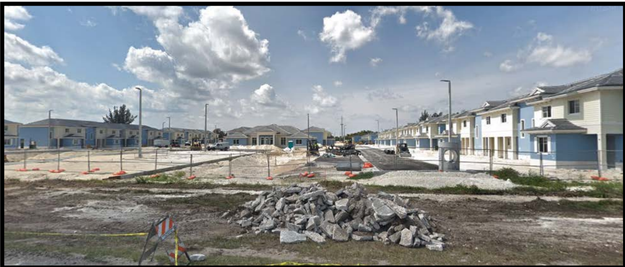
Apartments under construction (March 2019)
