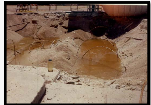
Tank removal excavation (1991)
