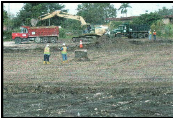
Soil and ash removal
