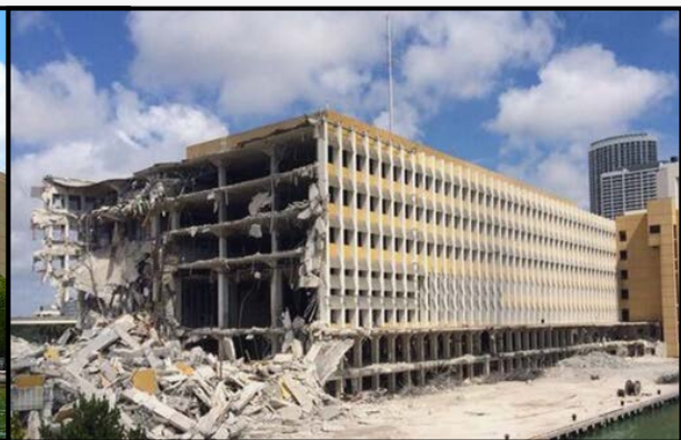
Demolition of Miami Herald Building (2014)
