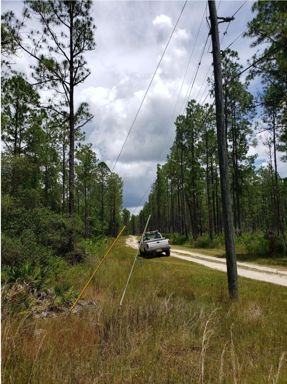
Photo – Power and existing forest road access located 300' southeast from development
