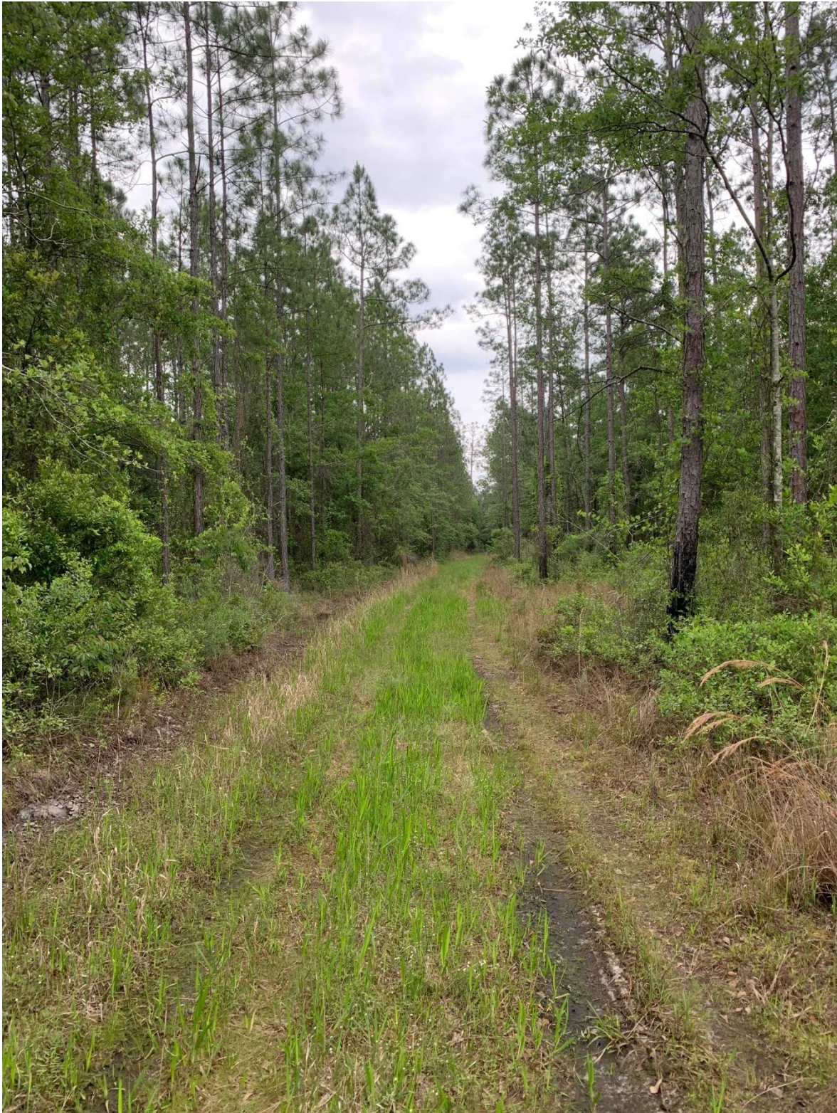
River Road Corridor Widening Beginning Point; Facing West from County Road 127
