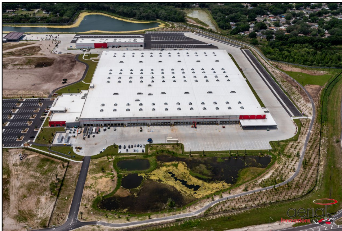
Above: Tilt-up walls May 2023 Left: Current construction progress April 2024
