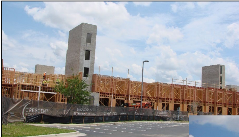
Left: Construction progress May 2023 Below: Construction progress September 2023
