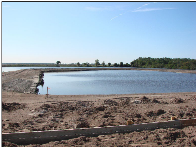
Left: Vapor barrier installation Above: Stormwater pond
