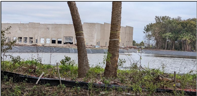
January 2022 construction of warehouse and lined pond
