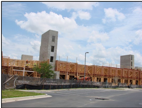
Above: Elevator towers and apartment framework in construction
