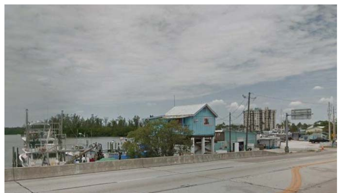
Pelican Bay Working Waterfront, Fort Myers Beach
