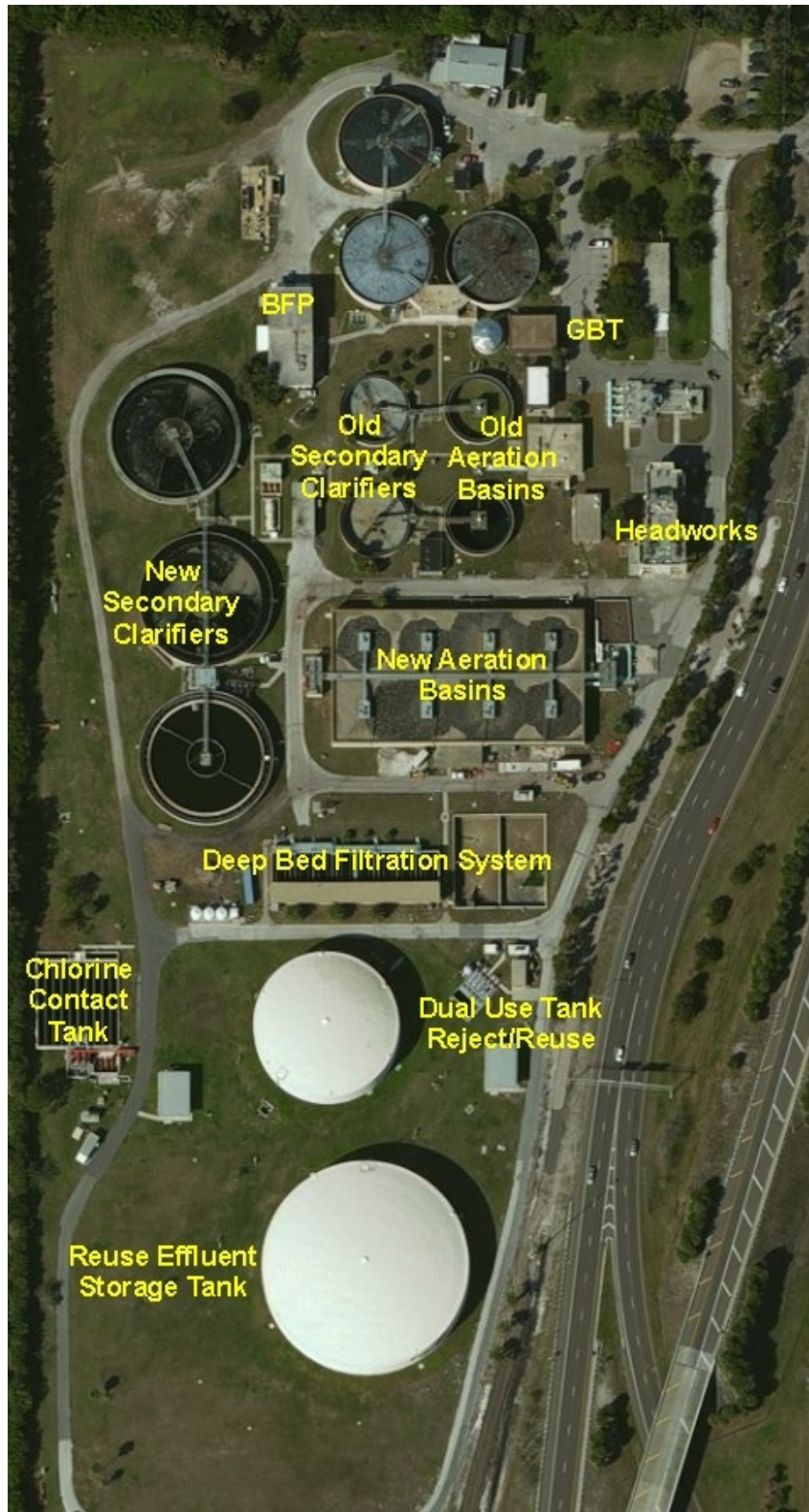
Figure 2-1. Aerial View of the SWWRF
