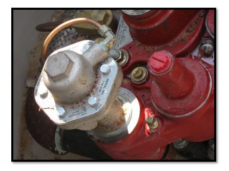
Pressurized small diameter piping in contact with the soil must be installed with line leak detectors, and must be tested for operability every 12 months.
