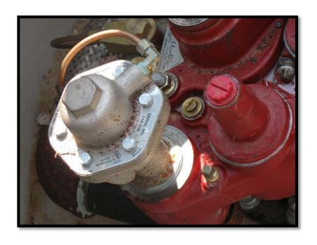
All new pressurized small diameter piping in contact with the soil must be installed with line leak detectors, and must be tested every 12 months.
