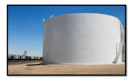
Field erected ASTs that are loaded by truck are required to have spill containment by July 11, 2017, unless the fill connection already exists within a dike field with secondary containment or within a tank truck containment area.
