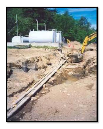
For new piping installed in contact with the soil, a survey drawing signed and sealed by a professional land surveyor or engineer must be completed and maintained.
