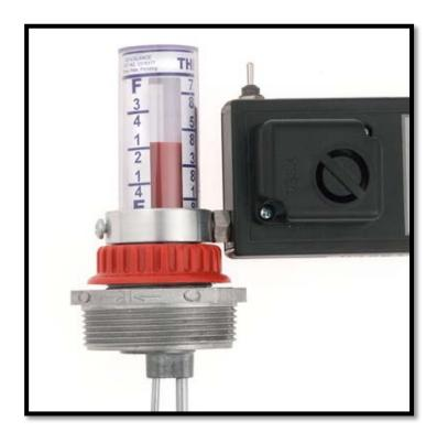
All overfill protection devices for ASTs must be tested for proper operation annually at intervals not exceeding twelve months. The initial testing must be conducted within 12 months of the effective date of the rule (by 1/11/18).
