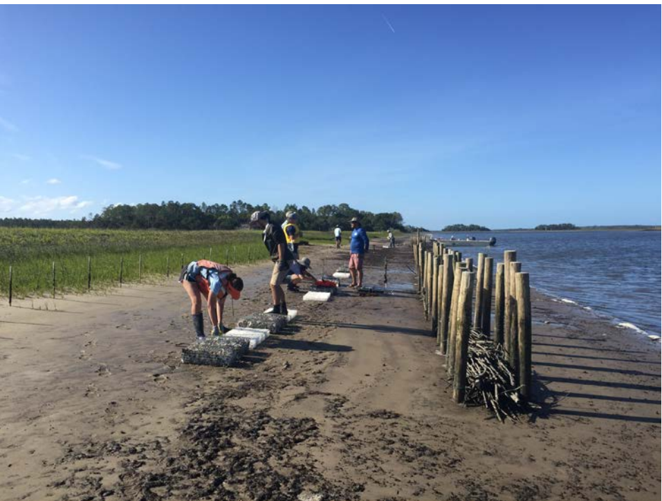
Experimental break walls and oyster restoration structures deployed at 6 high-energy sites within the GTM NERR, Ponte Vedra, FL
