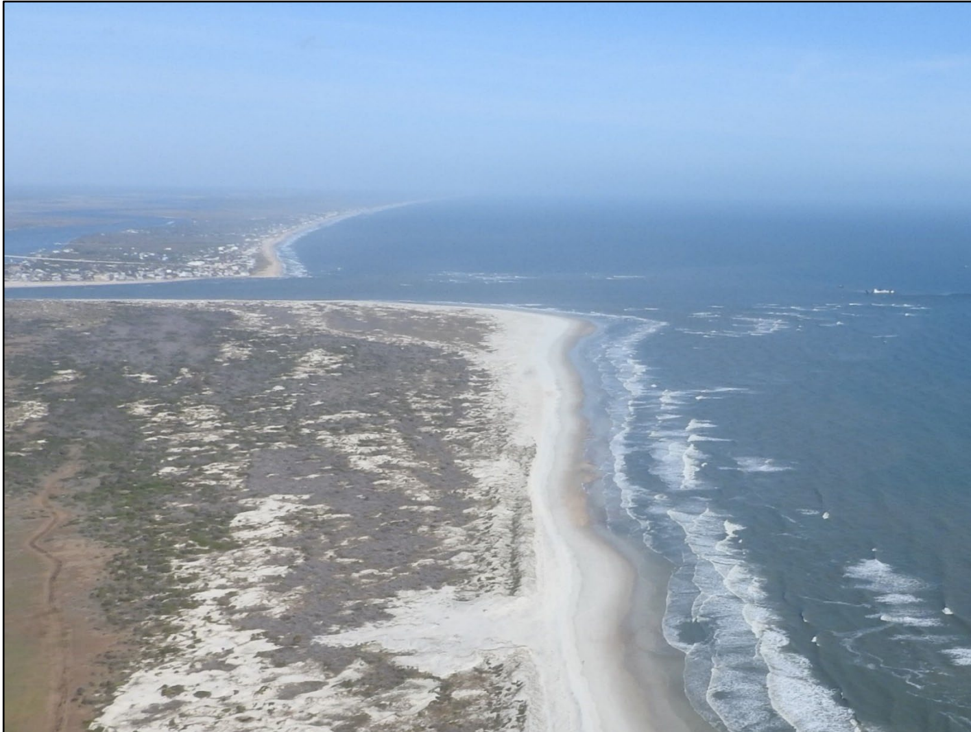
Figure 1: St. Augustine Inlet ebb shoal being dredged to bypass material south to construct the St. Augustine Beach nourishment project. Photo by Guy Weeks (DEP), February 2018.
