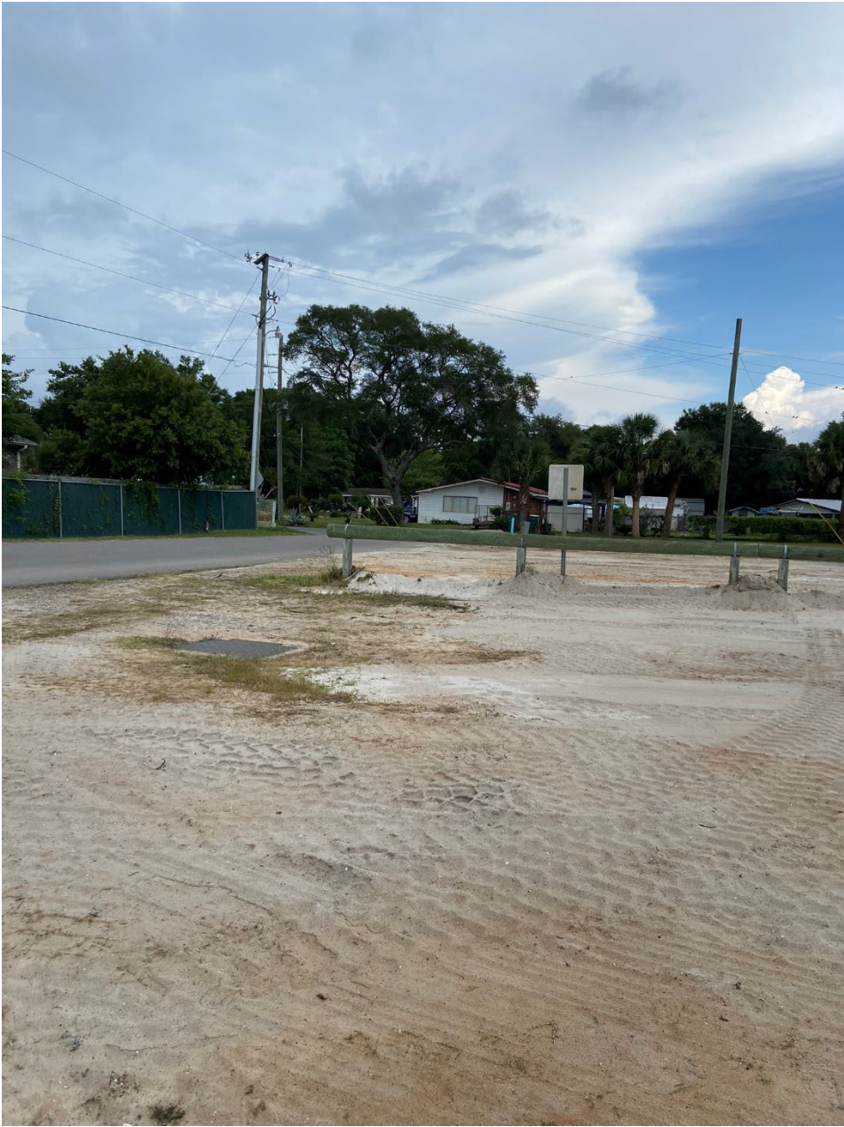
Figure 7.6 Sand pile removal East of FWB Stillwell Park Site (AQS # 12-091-0003)
