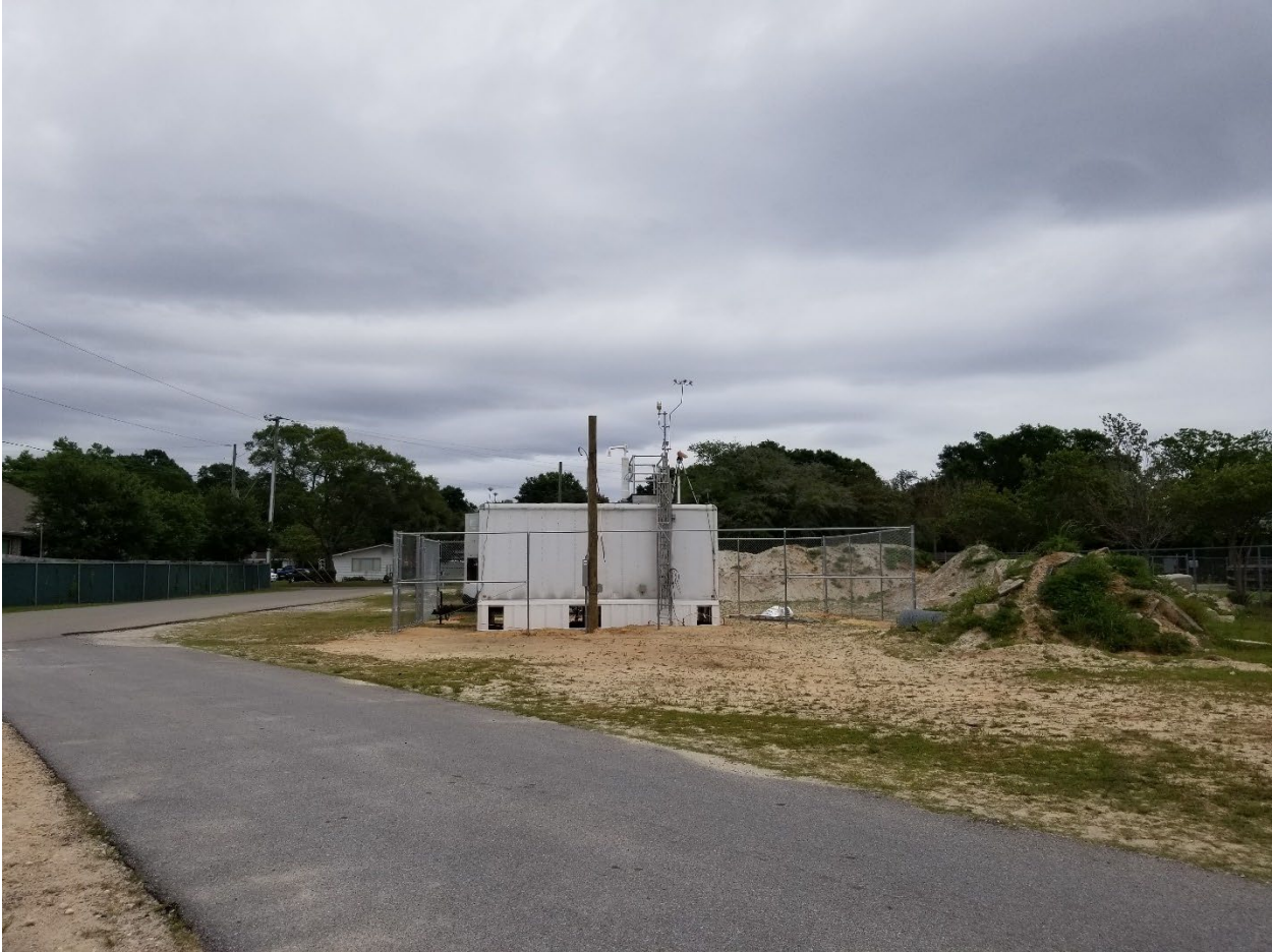
Figure 7.4 West from FWB Stillwell Park Site (AQS # 12-091-0003)
