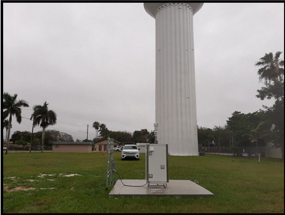
Figure 7.3 East from Wittkop Park Site (AQS # 12-086-6002)
