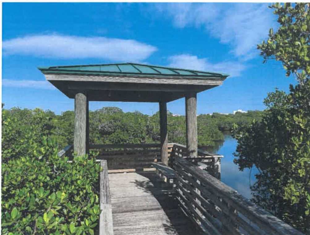
Photo 11 - Wildlife observation platform and access boardwalk. Looking north-northwest.
