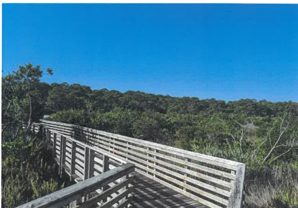
Photo 6 - Western portion of the boardwalk. Looking southwest.
