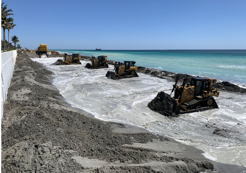
2020 Mid-Town Beach Nourishment – Palm Beach County Photo credit: Robert Weber, Town of Palm Beach
