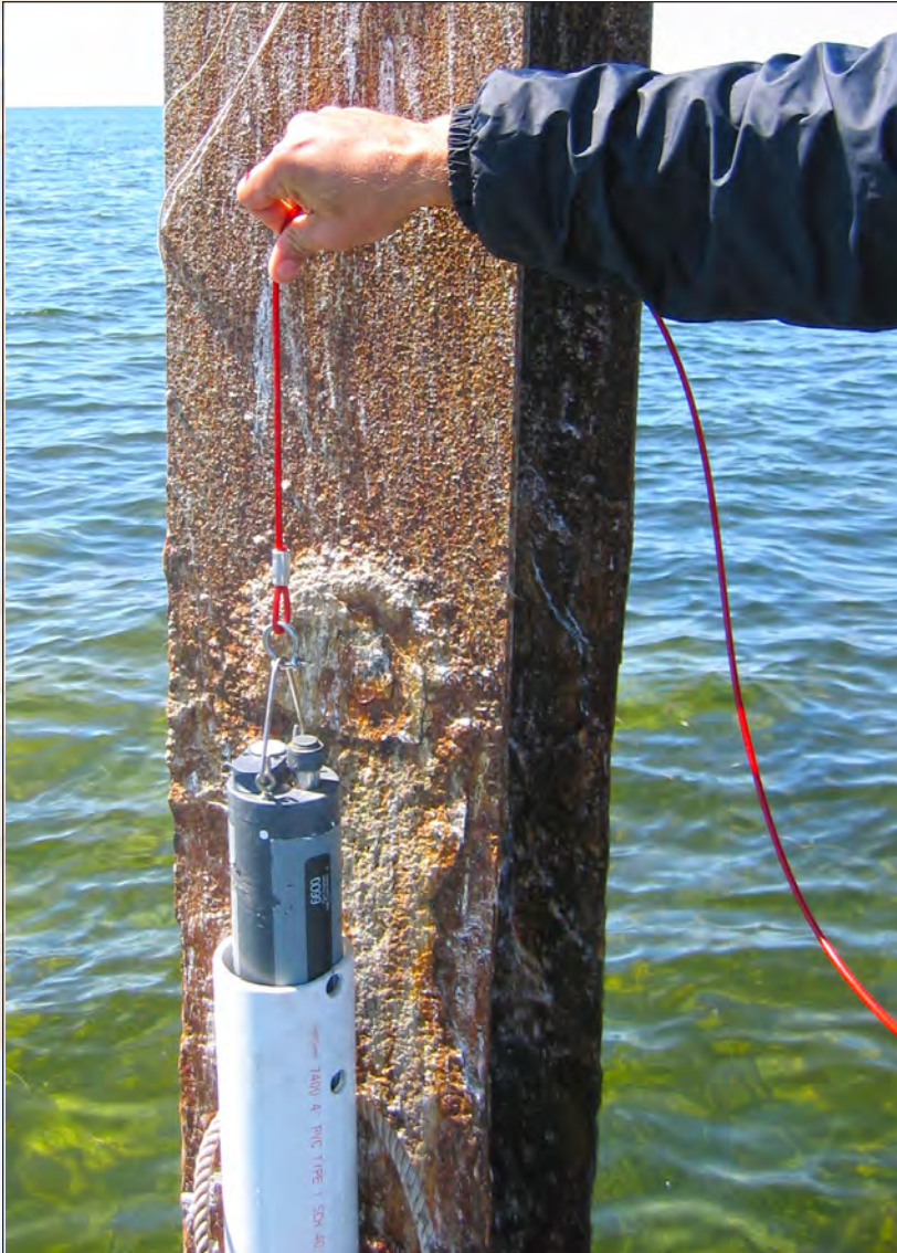
Water quality instruments are installed on navigational markers and must be maintained regularly by staff.
