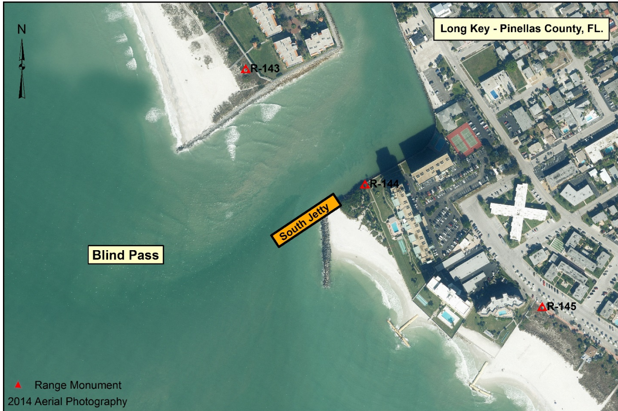
Figure 6. Graphic illustrating an extension of the south jetty as discussed in Alternative 5 (Wang et al., 2016).
