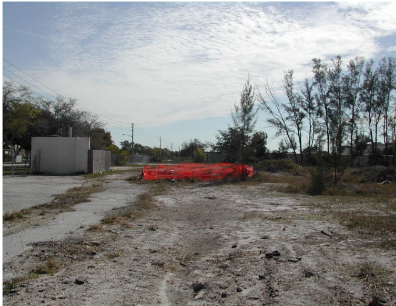
Above: The Pan American Brownfield Site in Coral Springs. The compound for the pump-and-treat remediation system is seen on the left.
