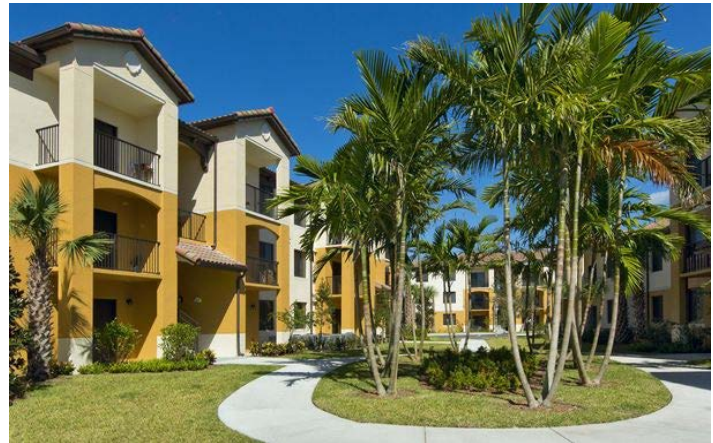
Above: Common space at Sorrento at Miramar as completed (taken November 2012)
