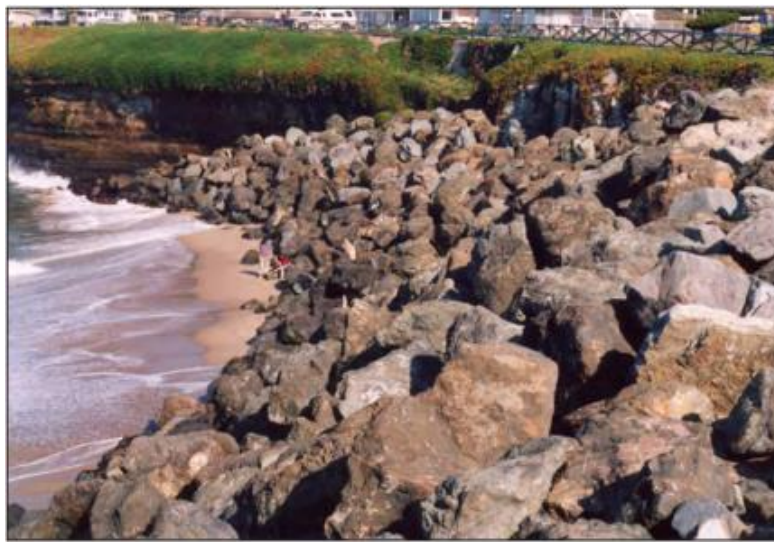
Figure 1. Revetment in Santa Cruz, California (note the absence of a sand beach). 11
