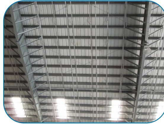
Reinforced Dry Stacks
