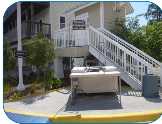
Fish Clean Table w/ signage
