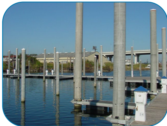
Pilings - 70 ft & 16 in Diameter
