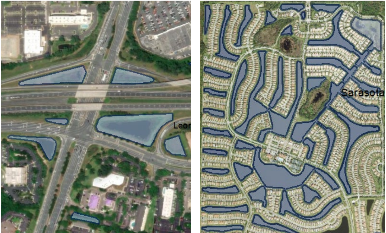
Figure 5. Stormwater treatment facilities: ponds coverage in Tallahassee, FL (left; roadway stormwater; 30.501960, -84.252182) and Venice, FL (right; subdivision stormwater; 27.041809, -82.342873)
