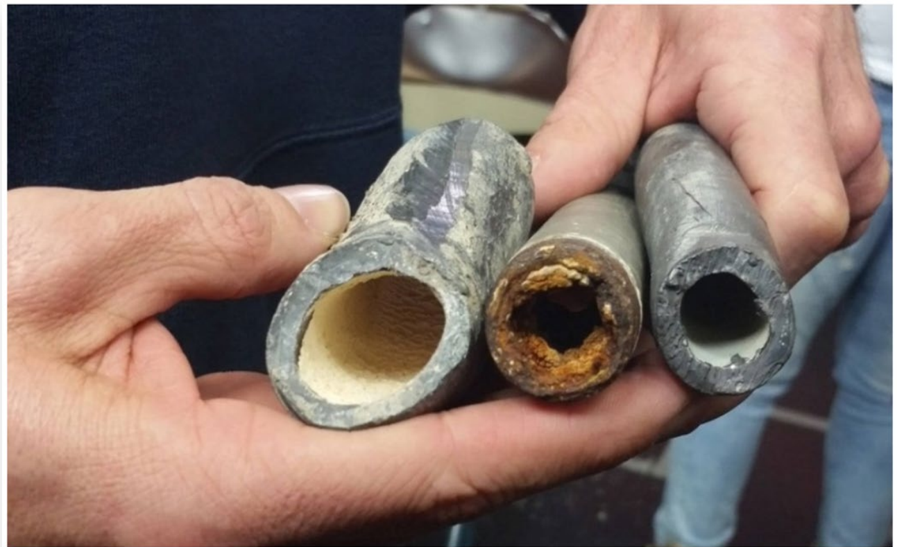
An EPA civil engineer shows how corrosion control treatments can affect lead pipes. The one on the left was treated, the middle one was not, and the one on the right is a new pipe. Lauren Chapman / IPB News, File Photo
