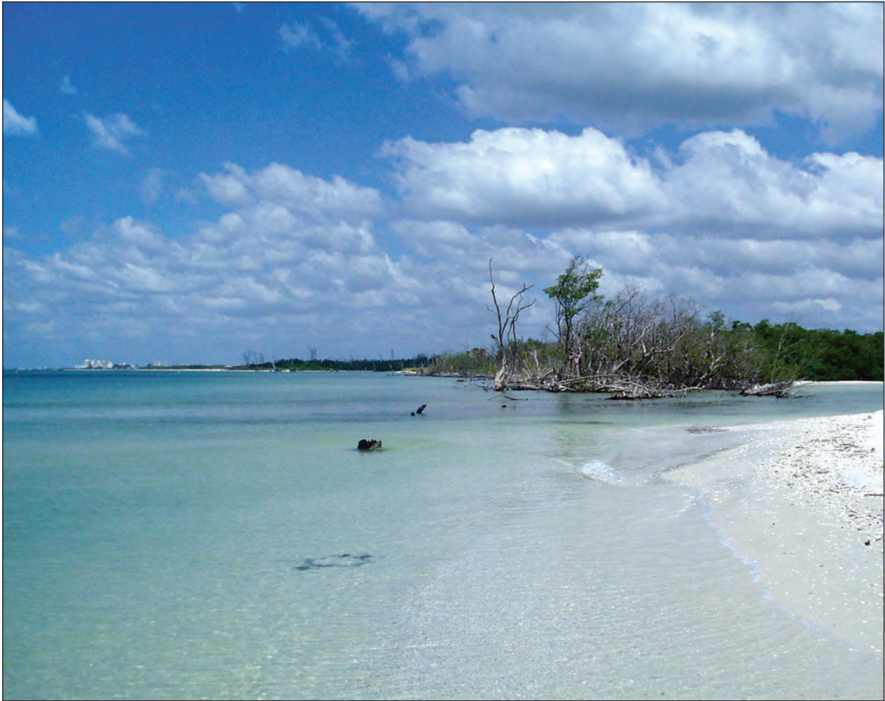
A bay-to-gulf breach through a barrier island leads to the pursuit of an erosion control project.
