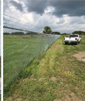
New Fencing and Signage Looking west
