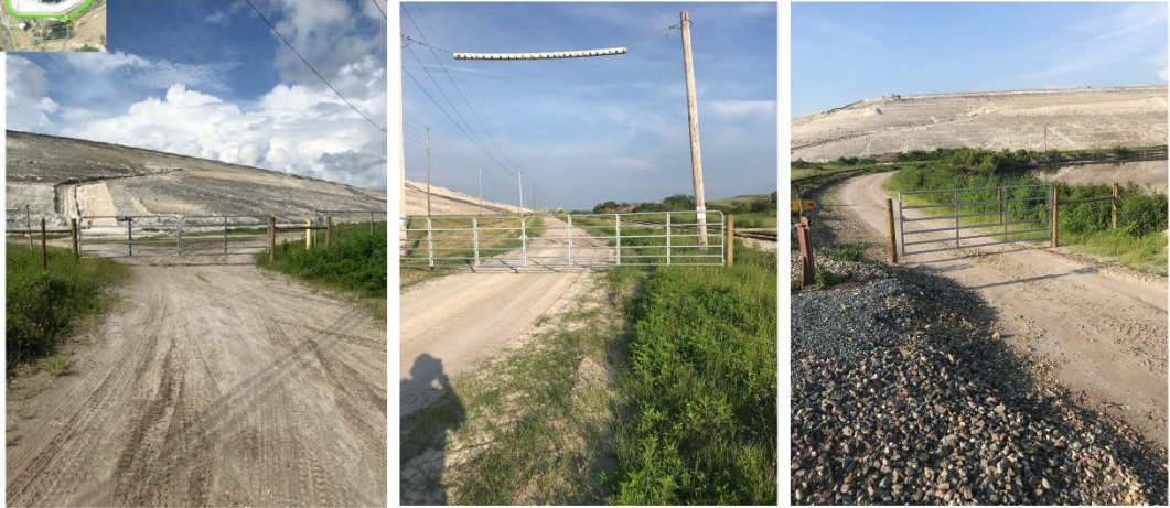
Locations No. 9 and 10 – Newly installed gates
