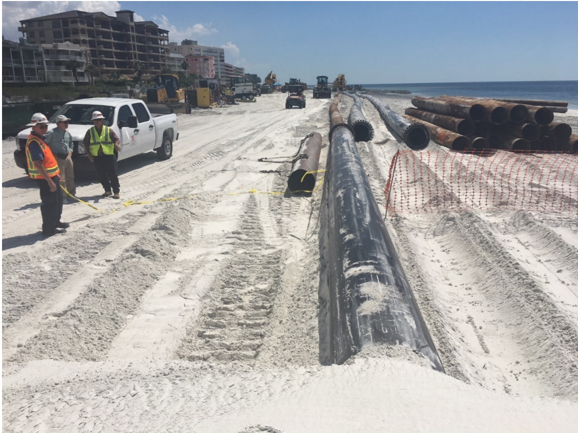
2018 Sand Key Segment – Pinellas County Shore Protection Project
