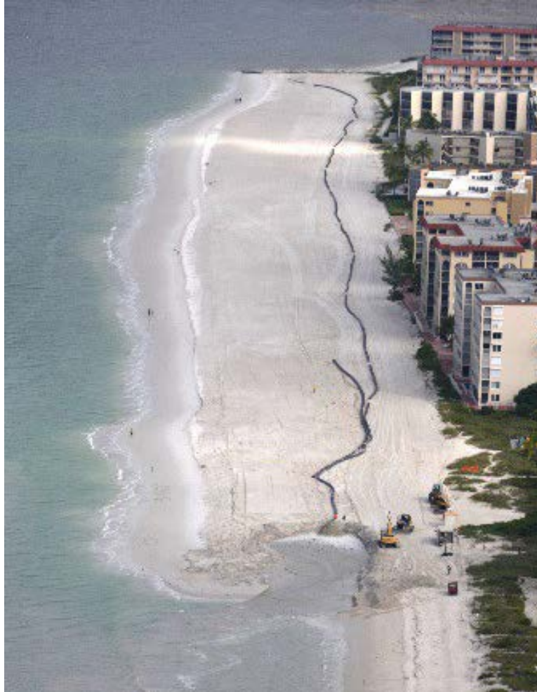
Bonita Beach Nourishment in 2014. Photo courtesy of Lee County.
