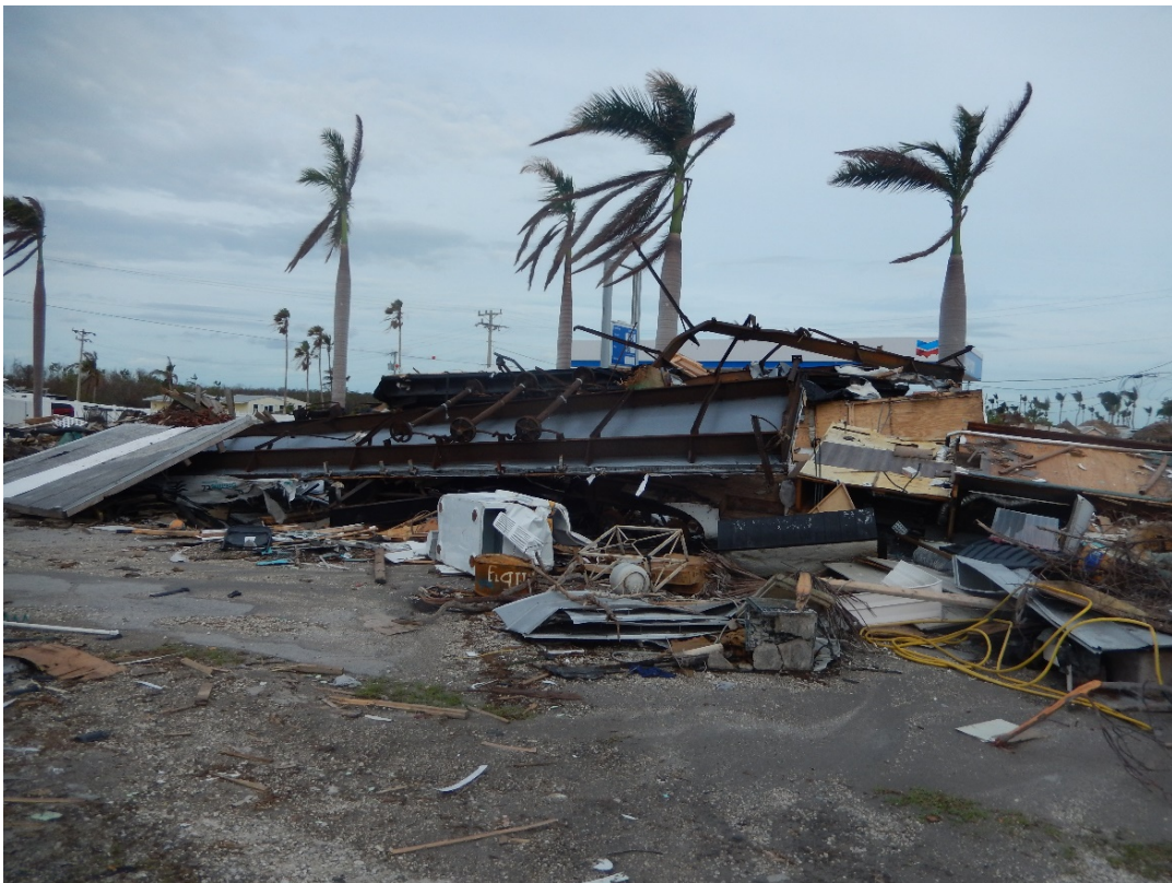
Figure 79. Trailer damage, Ohio Key Campgrounds.
