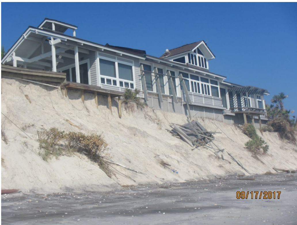
Figure 10. Major dune erosion threatening structure at R27.6, Ponte Vedra.
