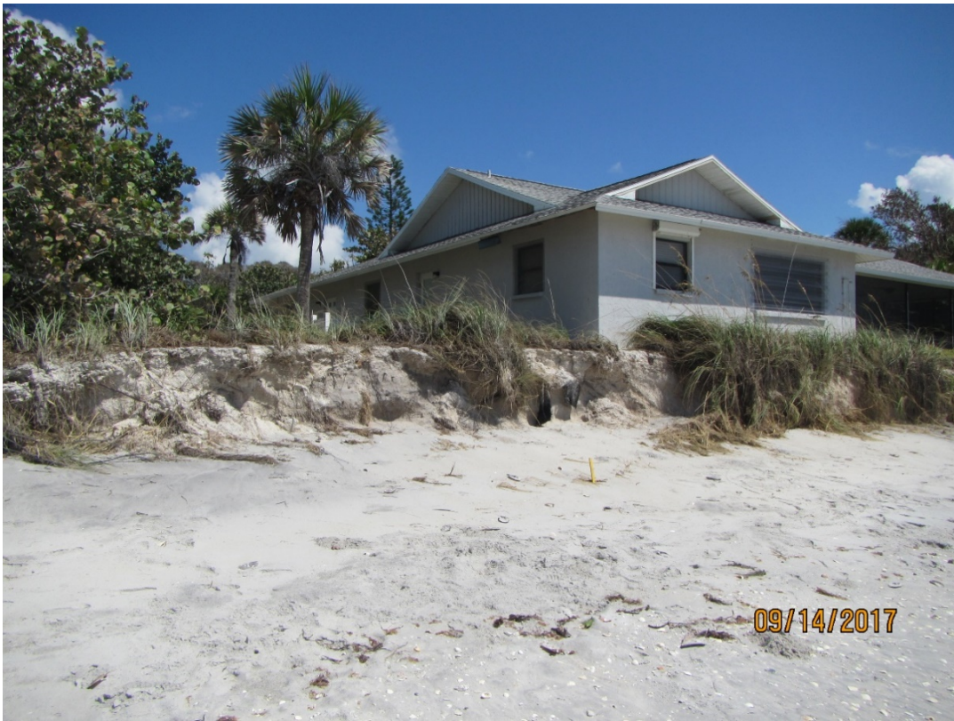
Figure 56. Dune erosion that threatened a residence near R182.
