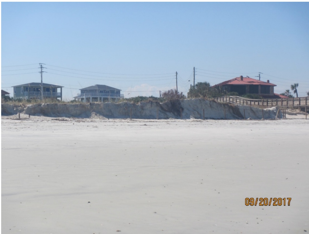
Figure 25. Major beach and dune erosion near R143, Town of Ponce Inlet.
