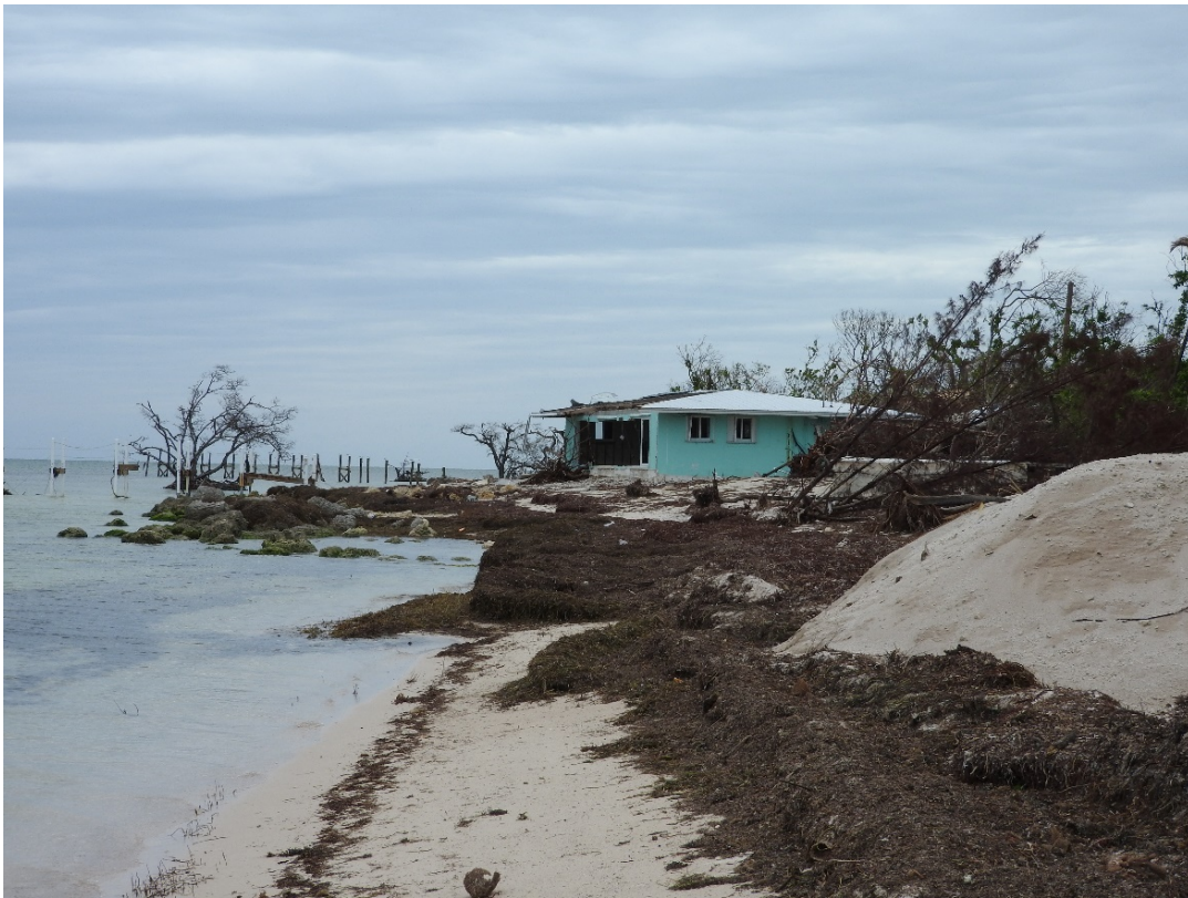
Figure 92. Dwelling and dock destroyed, Long Beach, Big Pine Key.
