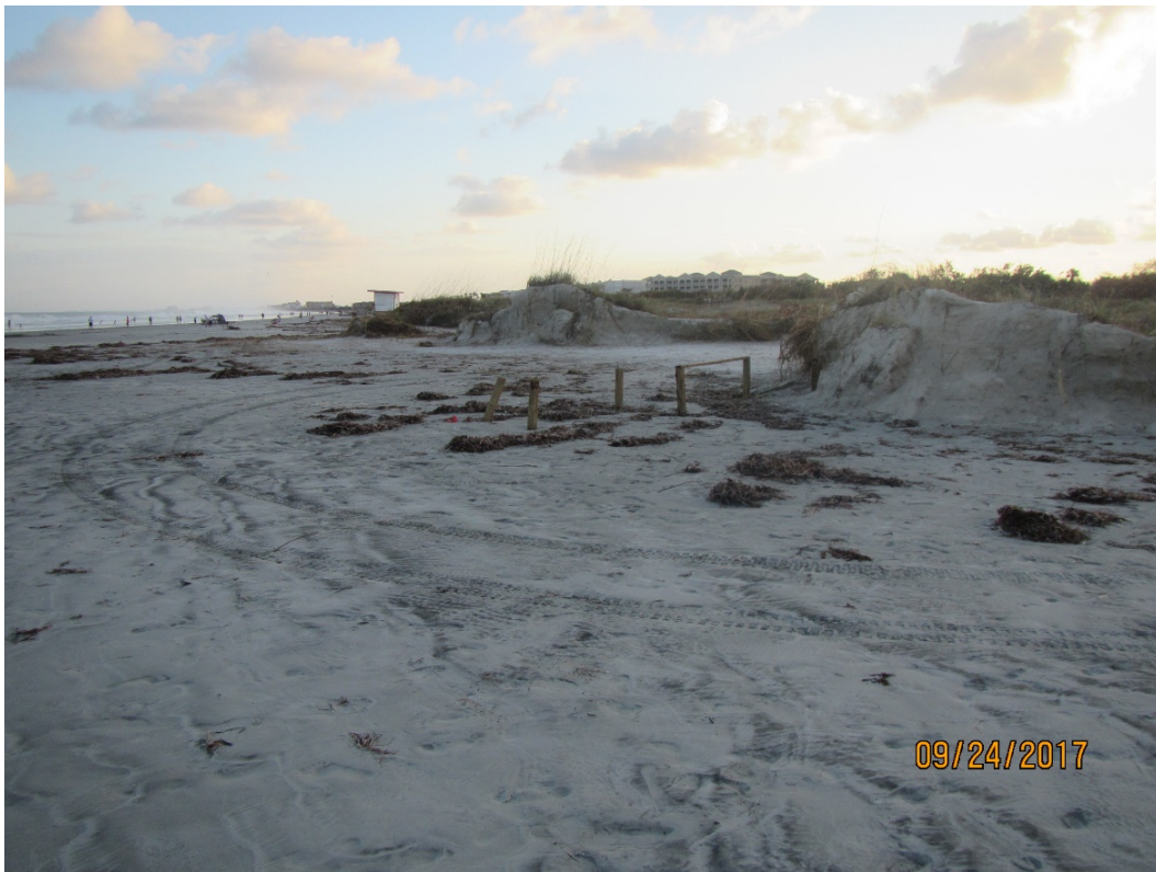
Figure 30. Major dune erosion at Jetty Park near R1, Port Canaveral.
