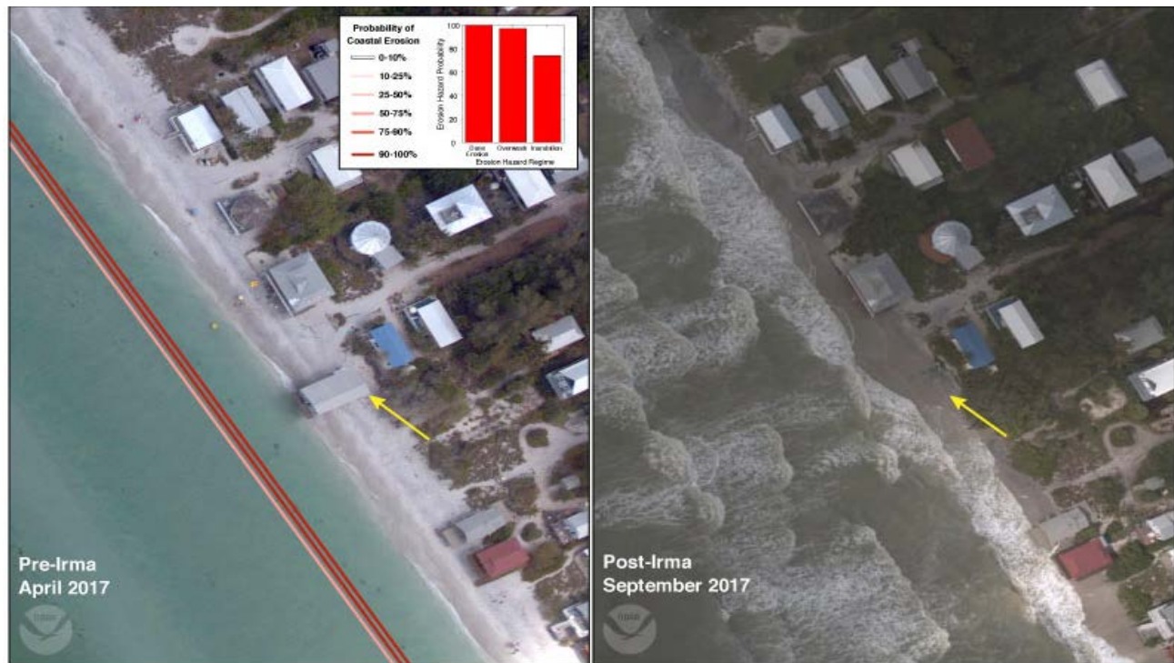
Figure 53. Comparative NOAA aerial photos showing the dwelling on Little Gasparilla Island destroyed near R49 (Source: National Assessment of Coastal Change Hazards, St. Petersburg Coastal and Marine Science Center, USGS).
