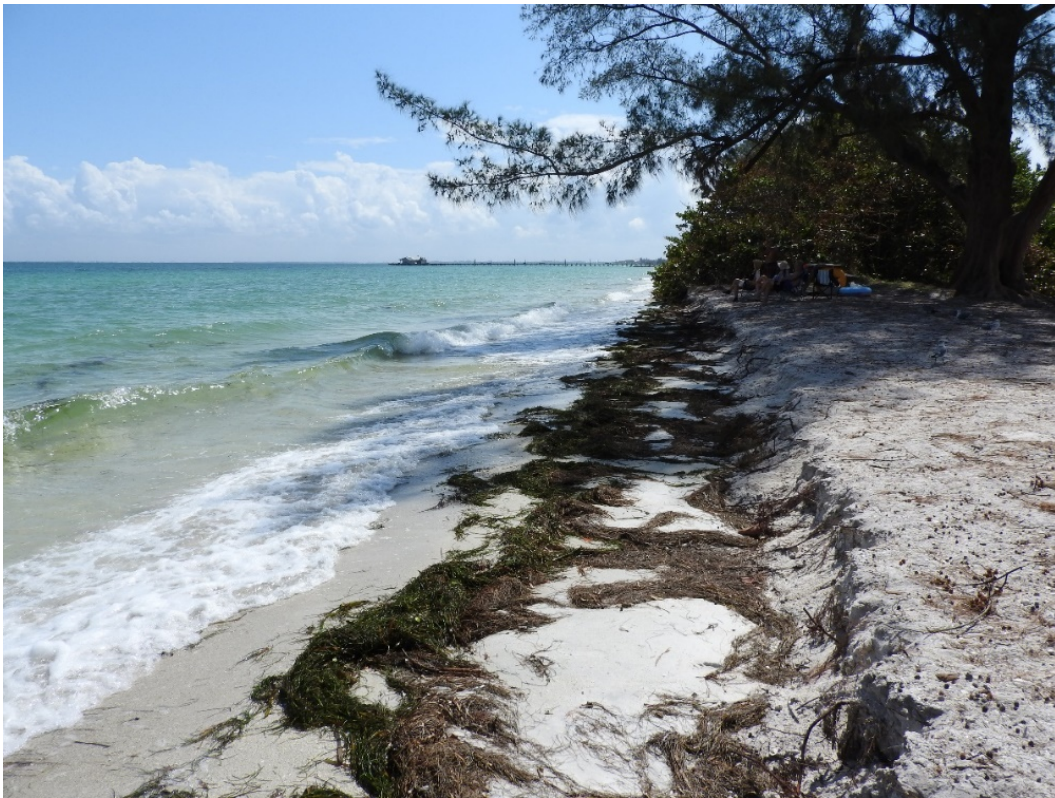
Figure 58. Beach erosion at the northern end of Anna Maria Island between R2 and City Pier.
