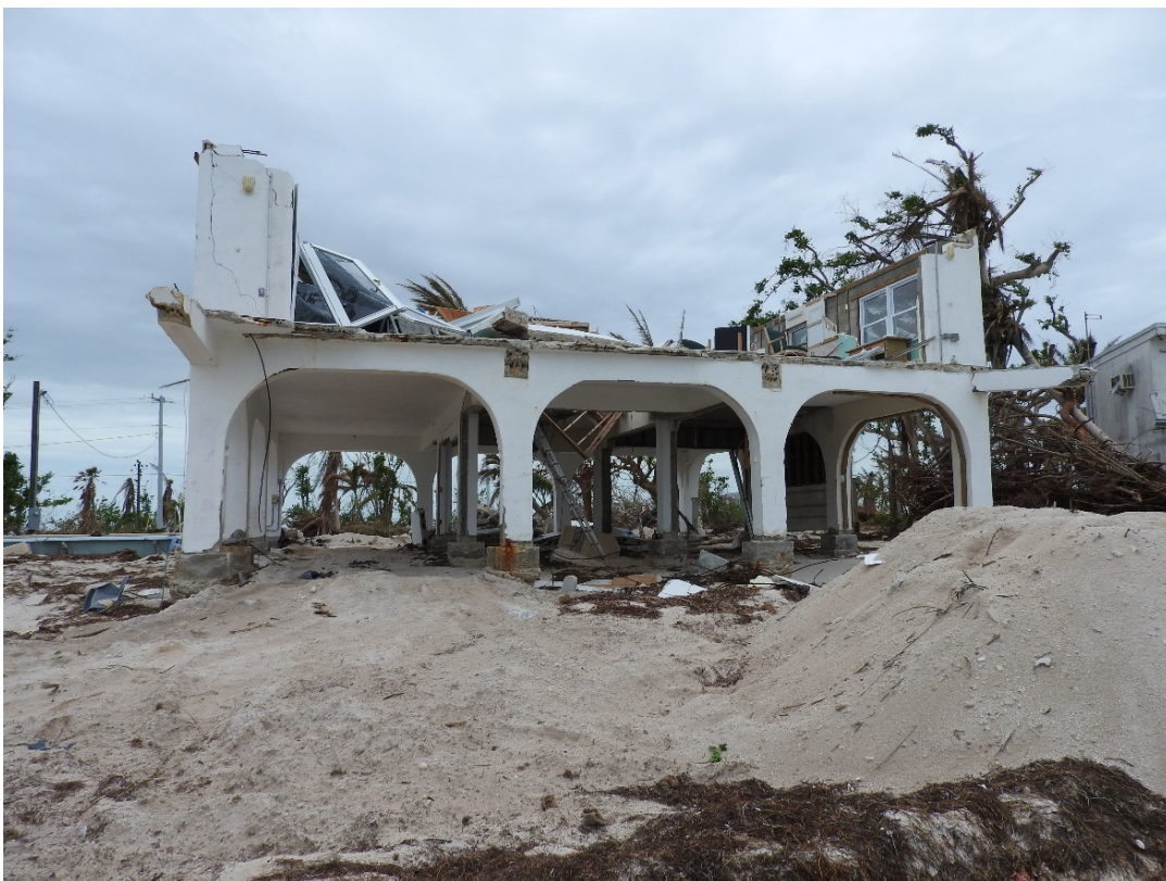
Figure 91. Single-family dwelling destroyed, Long Beach, Big Pine Key.
