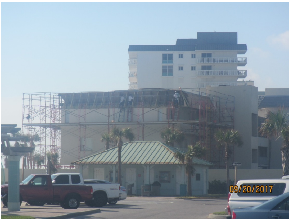
Figure 27. Wind damage to condominium at R40, Ormond Beach.
