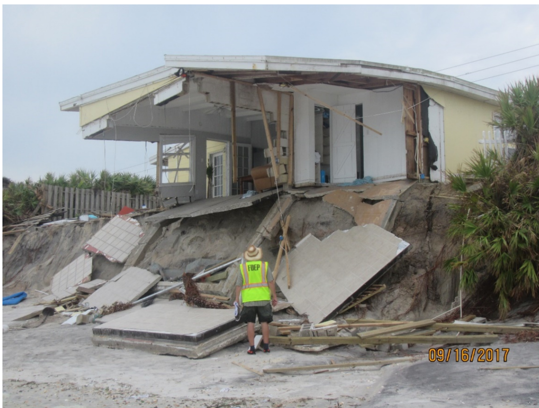
Figure 16. Single-family dwelling destroyed near R94, South Ponte Vedra.
