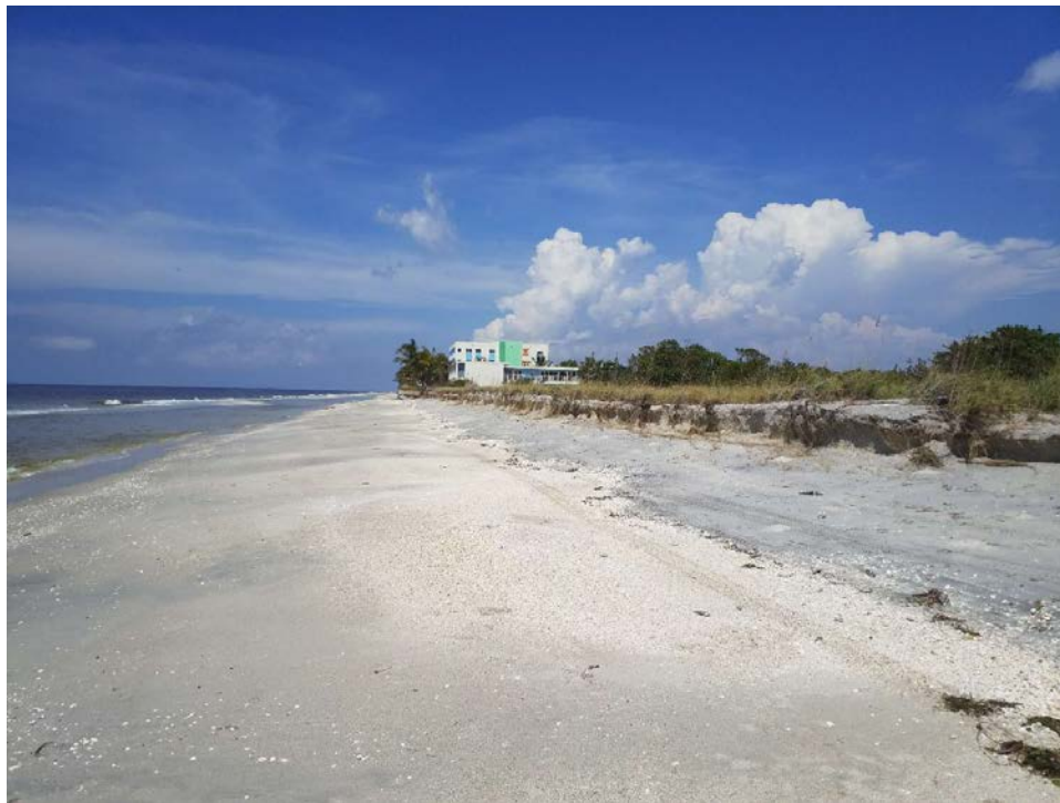
Figure 52. Beach and dune erosion at Stump Pass State Park near R16.
