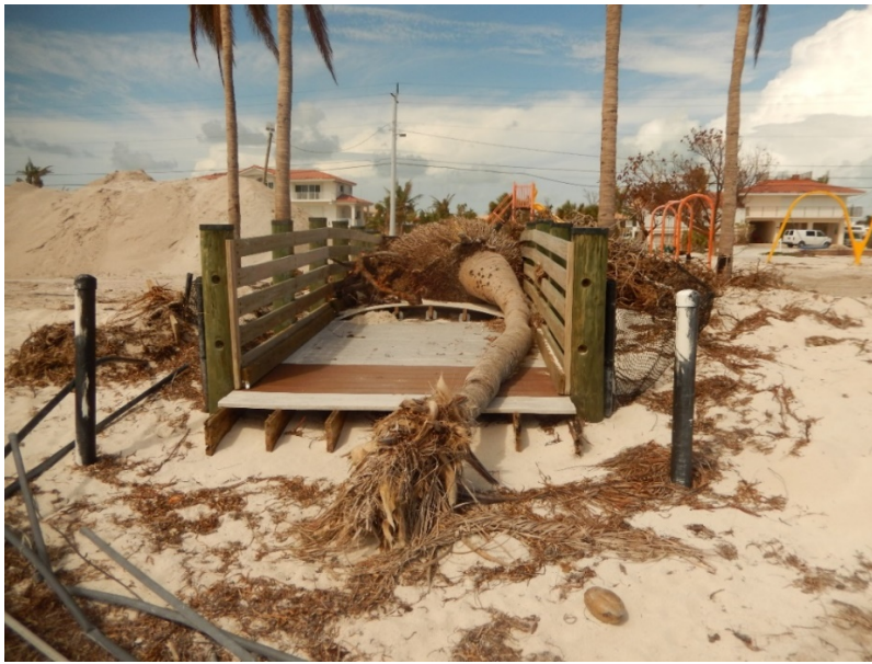
Figure 74. Damaged walkway and dunes, Sombrero Beach.
