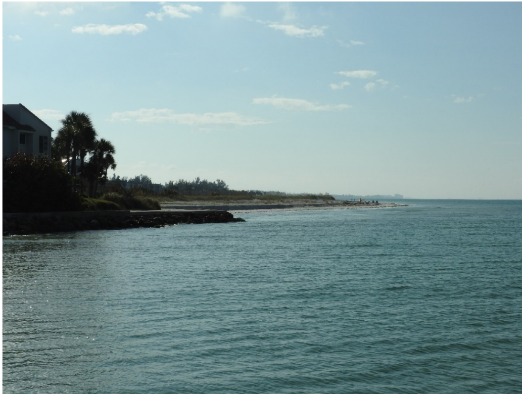
Figure 59. The northern end of Longboat Key had severe erosion between R43 and R45.
