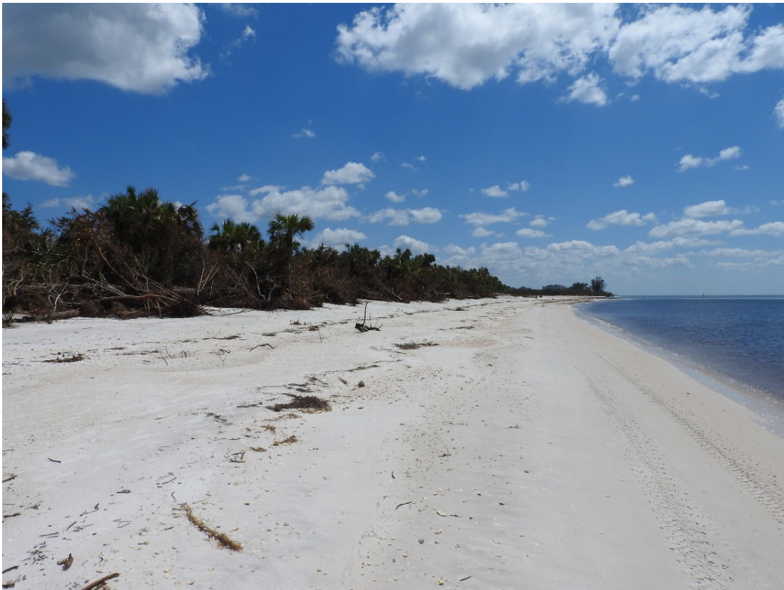
Figure 40. Major beach and dune erosion near R15 north of Wiggins Pass looking south.
