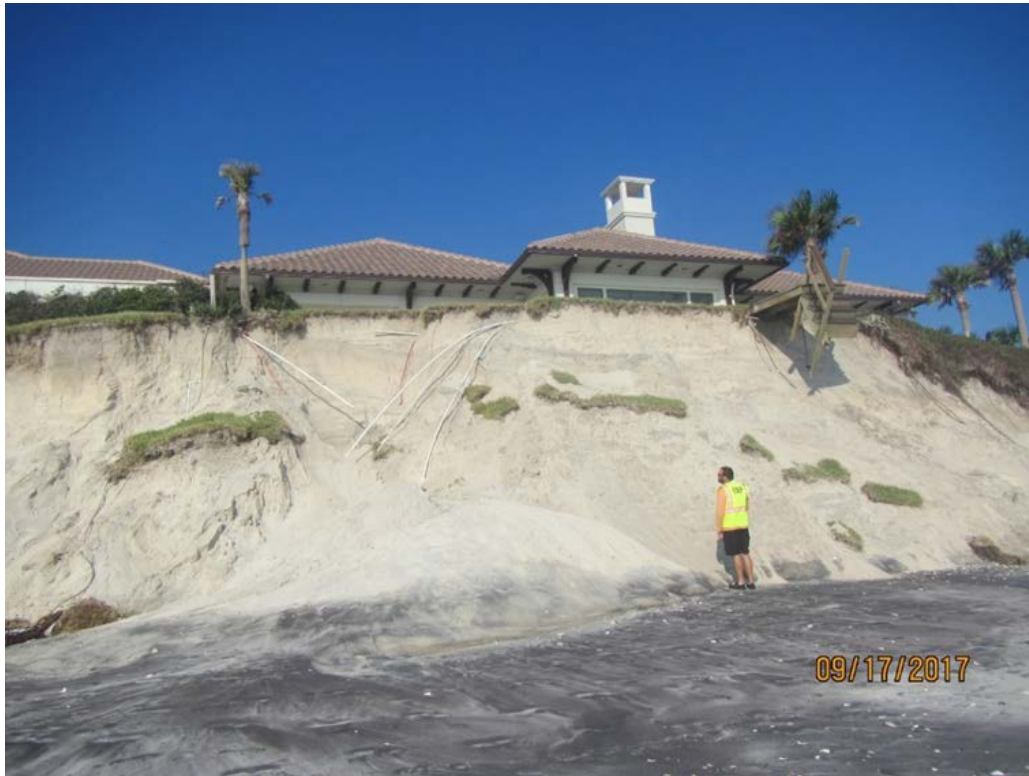
Figure 9. Major dune erosion threatening structure at R30, Ponte Vedra.
