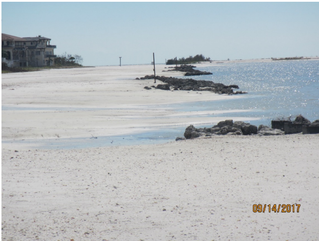
Figure 38. T-groin field along Hideaway Beach near V313.
