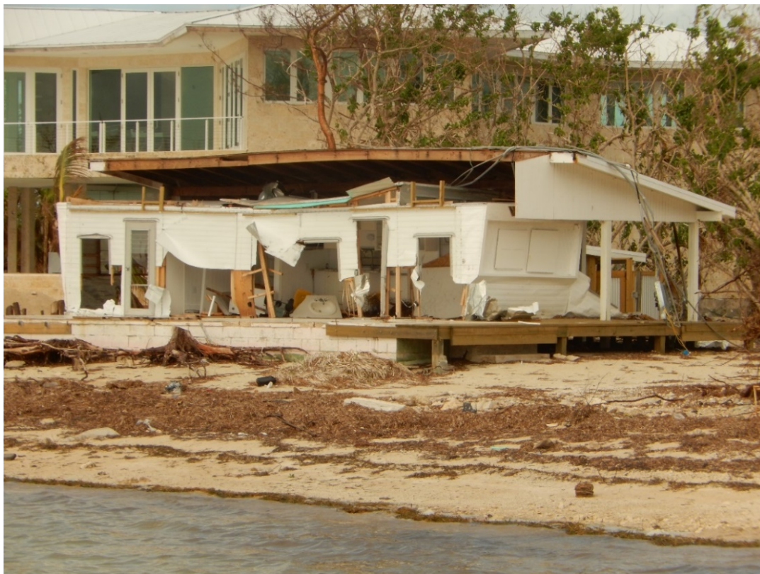
Figure 65. Single-family dwelling destroyed on Grassy Key.
