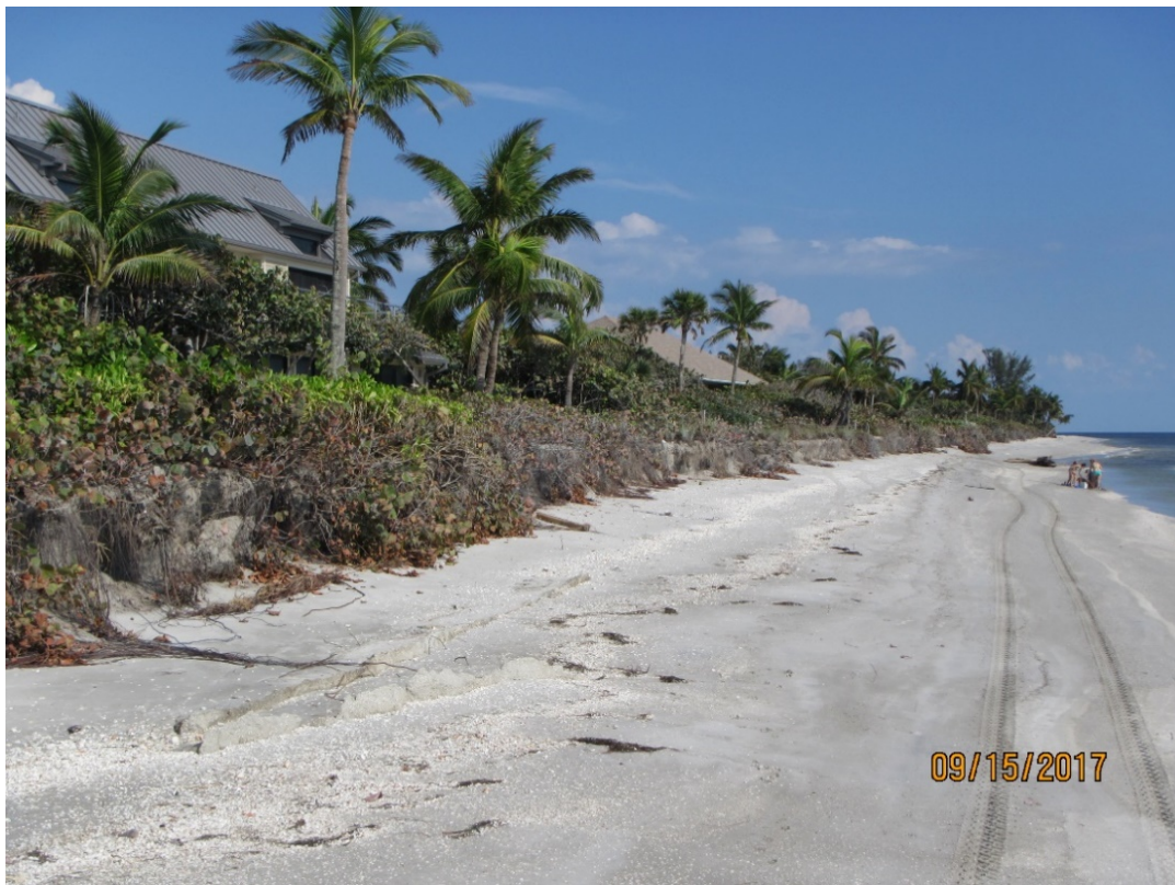
Figure 46. Erosion at the southern end of Sanibel Island near R131.
