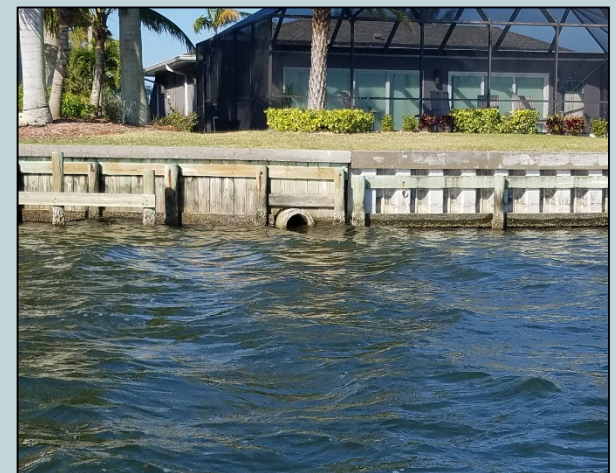
Bulkhead with outfall
