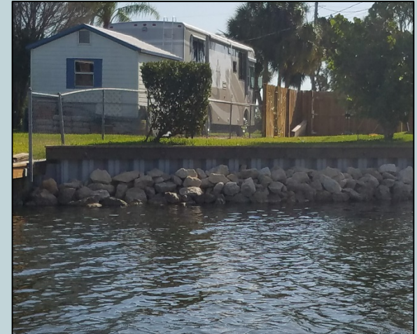
Bulkhead with Rip-Rap
