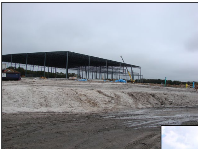
Warehouse construction over fill
