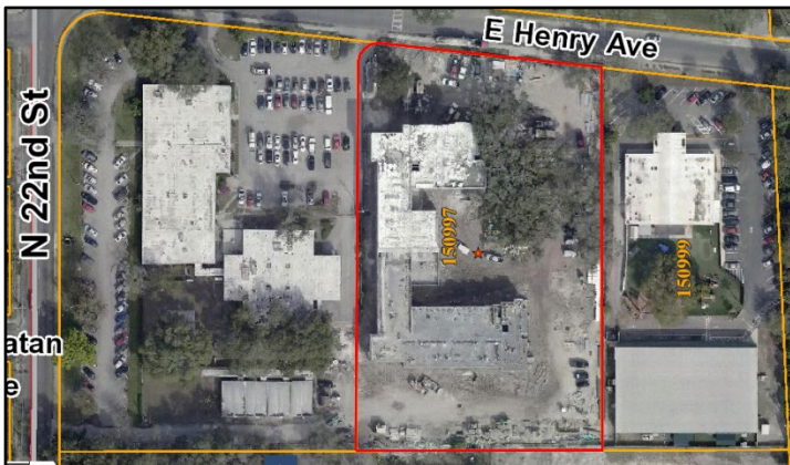
Aerial view of site prior to redevelopment. Site is currently under construction.
