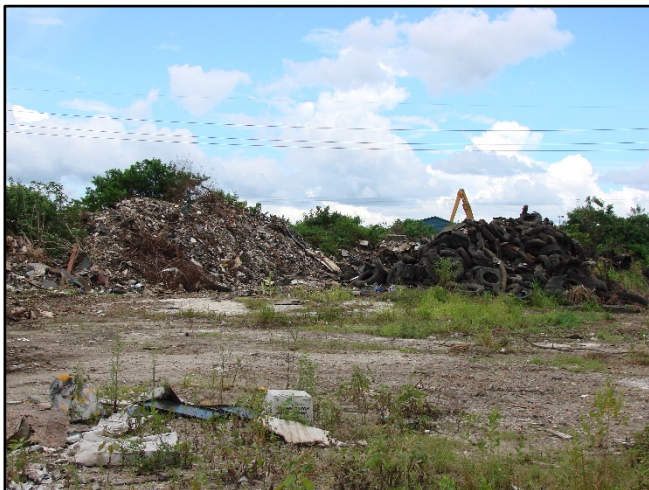
Piles from sorted surface debris. Some waste recycled.
