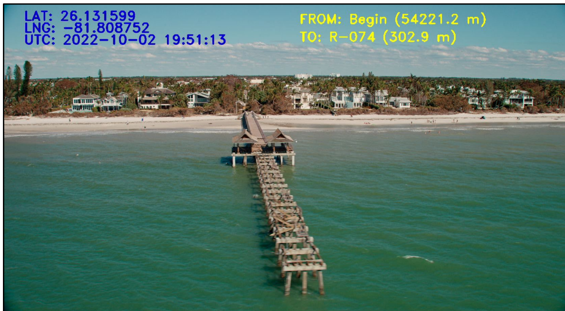
Figure 51. Damage to the Naples Pier (R-74).
