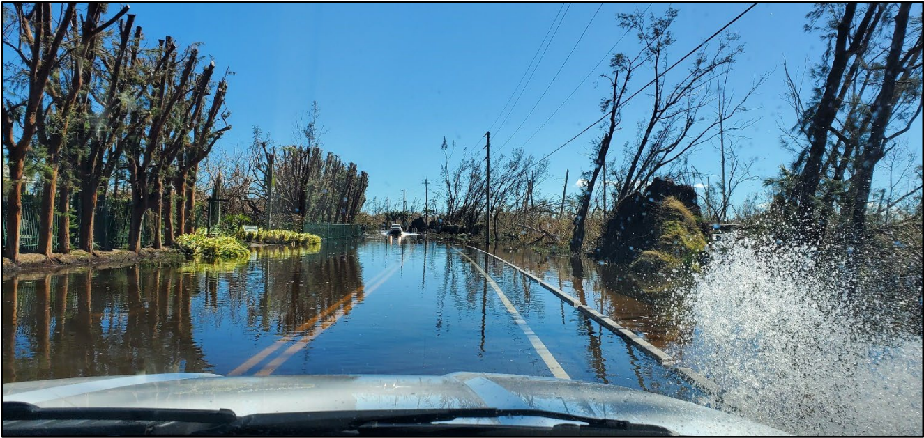
Figure 24. Storm surge and rainfall flooding on northern Gasparilla Island (R-61).
