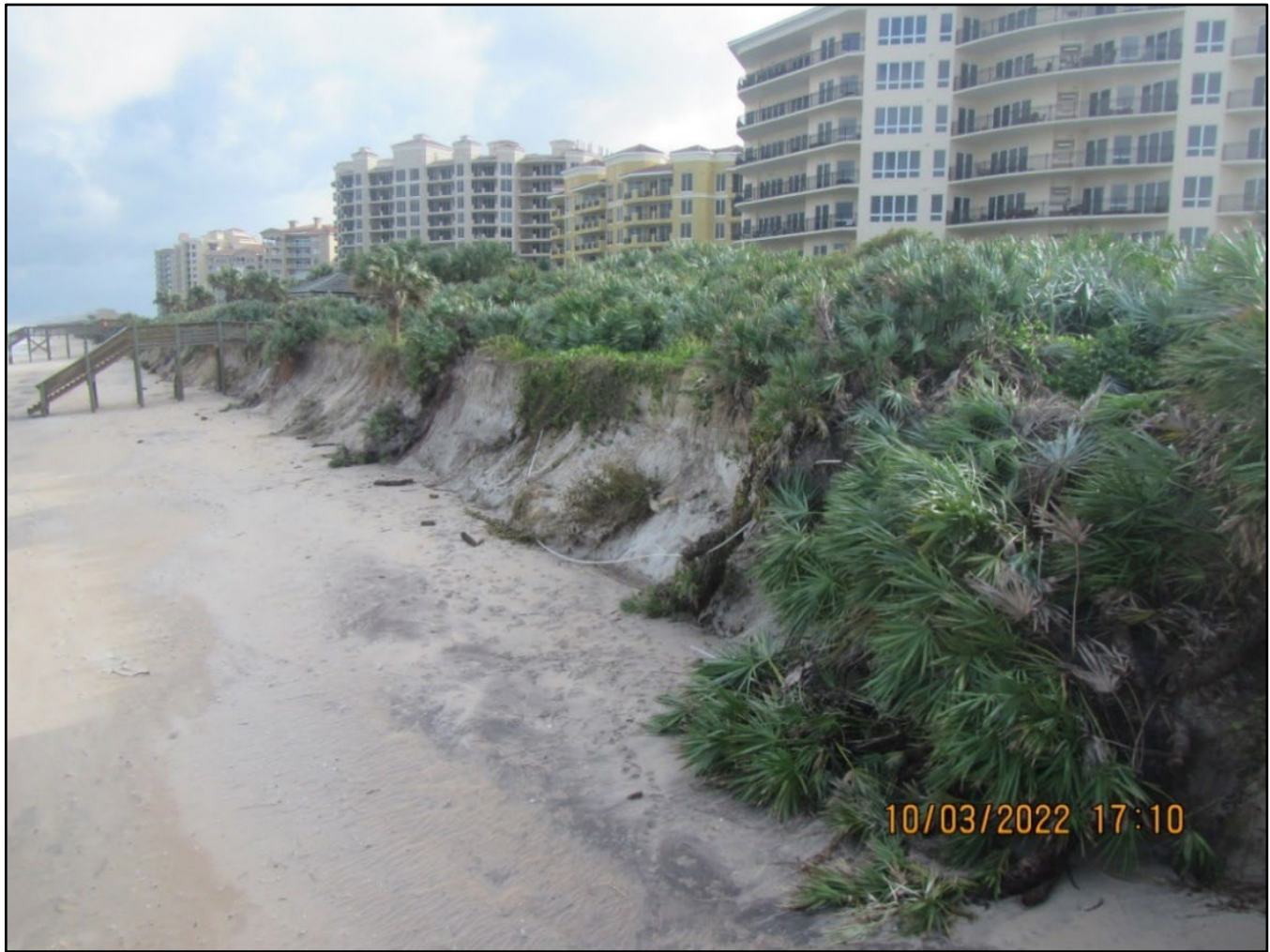
Figure 72. Major beach and dune erosion at Ocean Hammock after Hurricane Ian (R-38).
