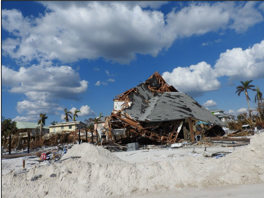
Figure 44. Single-family dwelling destroyed at Ft. Myers Beach near Lazy Way (R-196).
