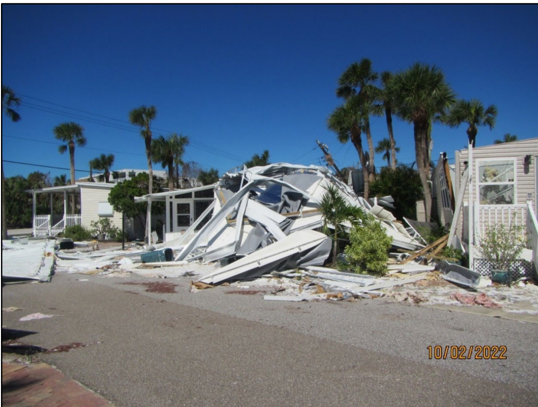
Figure 23. Mobile homes destroyed at Englewood Beach on Manasota Key (R-9).
