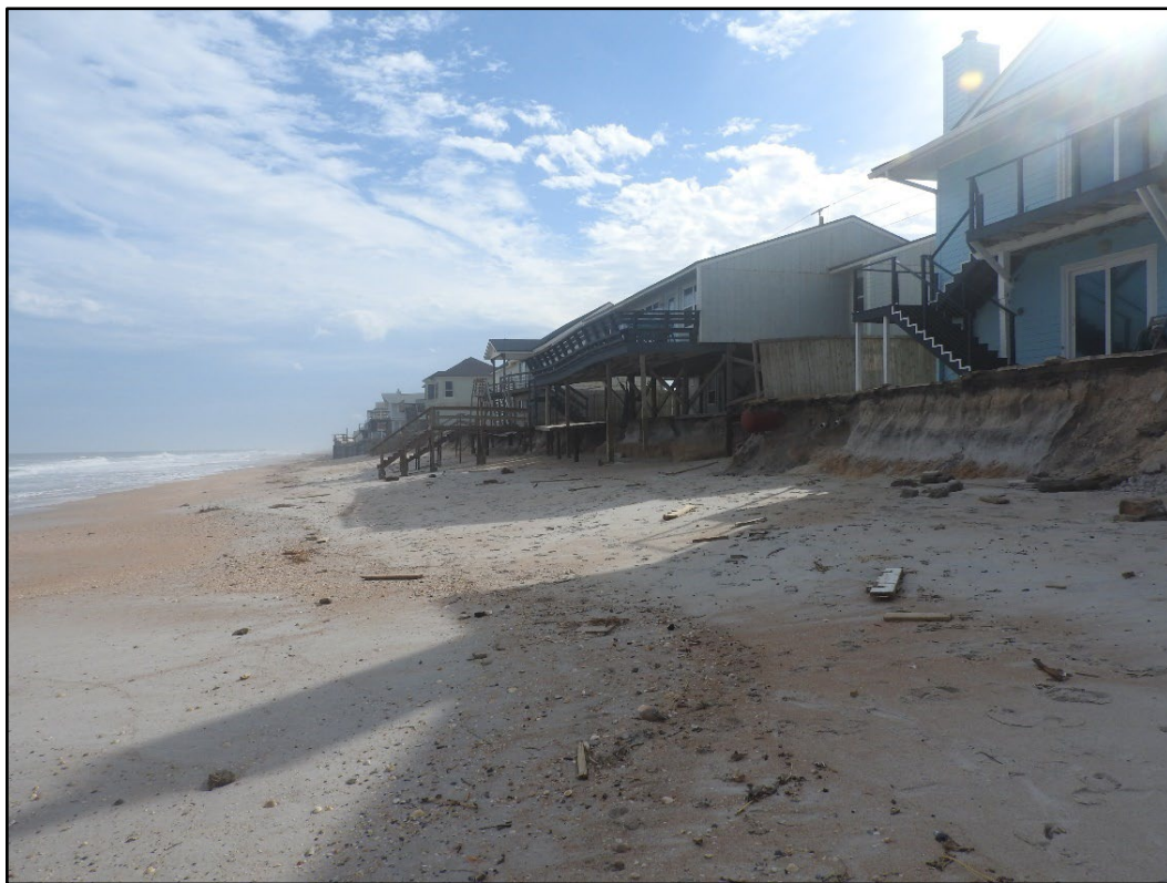
Figure 57. Major beach and dune erosion in South Ponte Vedra Beach (R-86).
