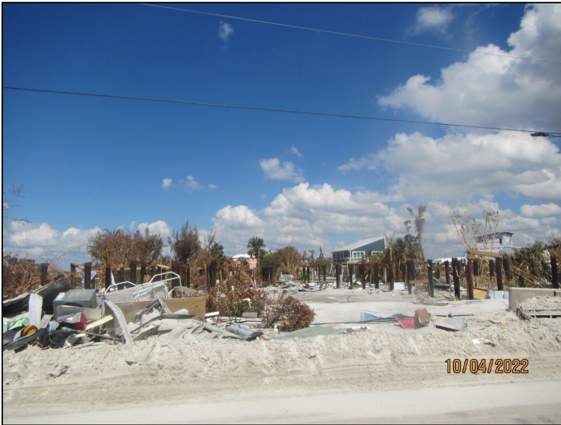
Figure 43. Homes destroyed and removed off pilings, Ft. Myers Beach near Matanzas St. (R-179).
