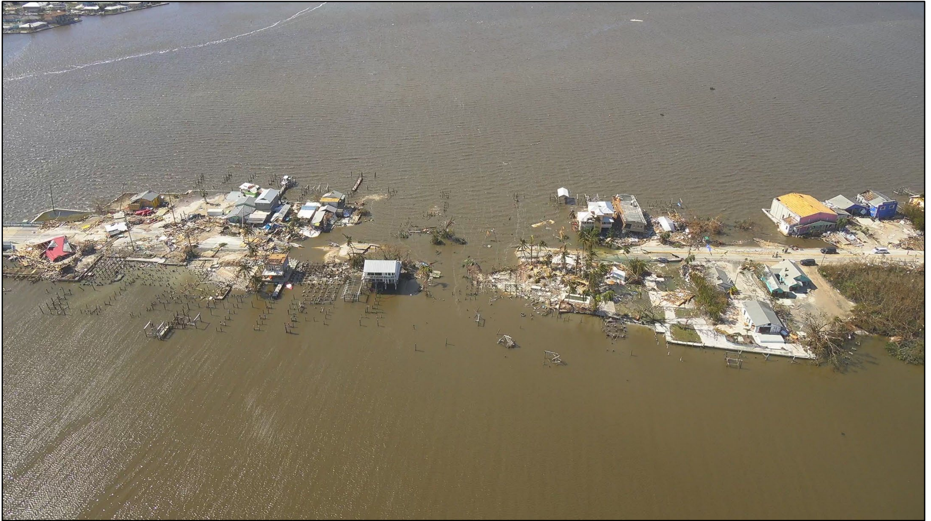
Figure 36. Pine Island causeway destroyed. Photo courtesy of Florida State University - Emergency Management and Homeland Security Program/ Florida UAS-1. Photo taken on September 29 th , 2022.
