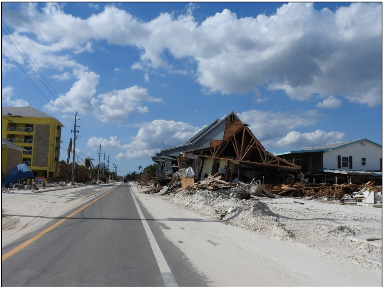
Figure 39. Storm surge transported Lahaina resort structures across Estero Blvd. (R-196).
