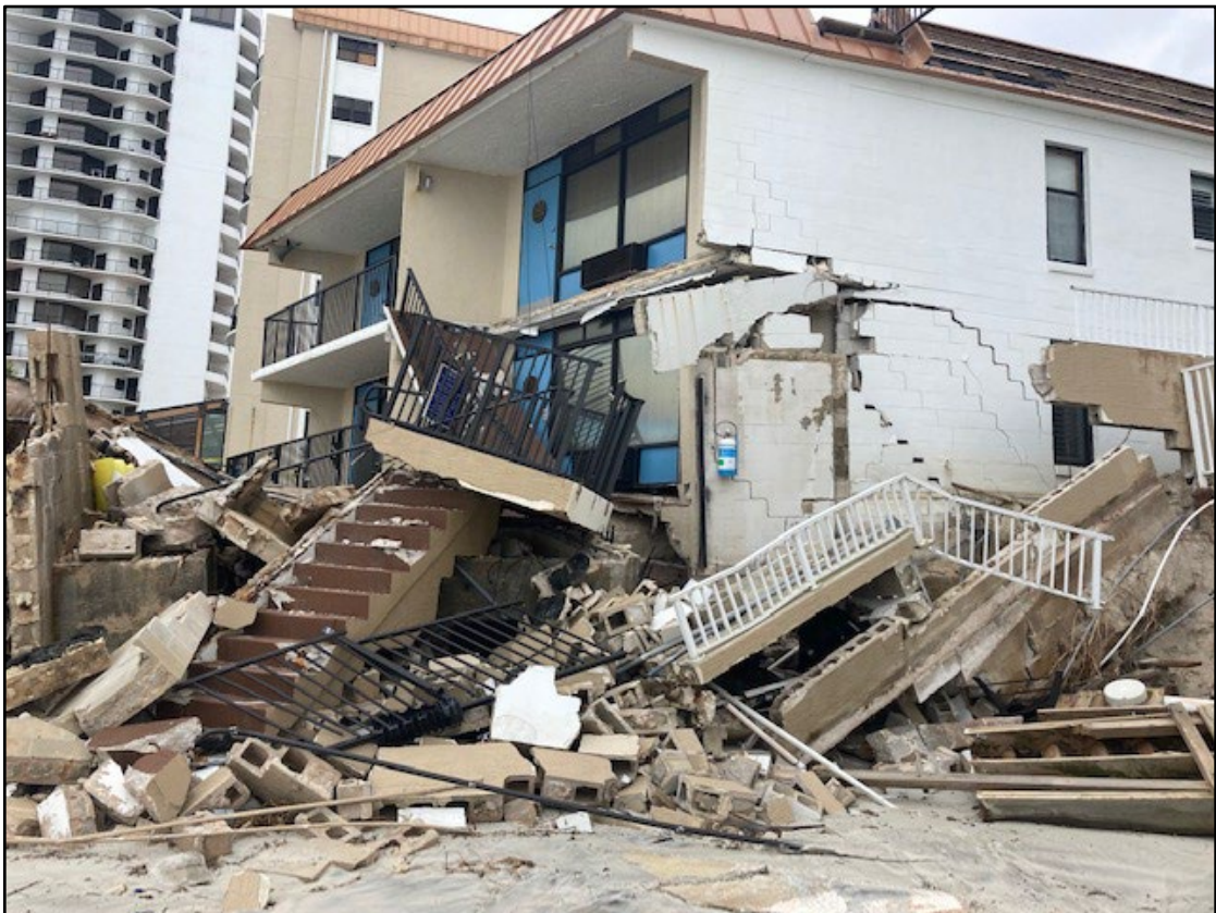
Figure 118. Damaged multifamily dwelling in Volusia County.
