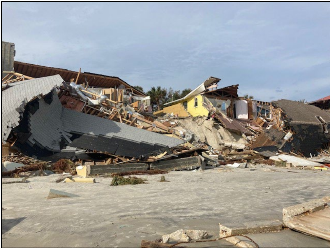
Figure 111. Homes destroyed, Wilbur-by-the-Sea (R125).
