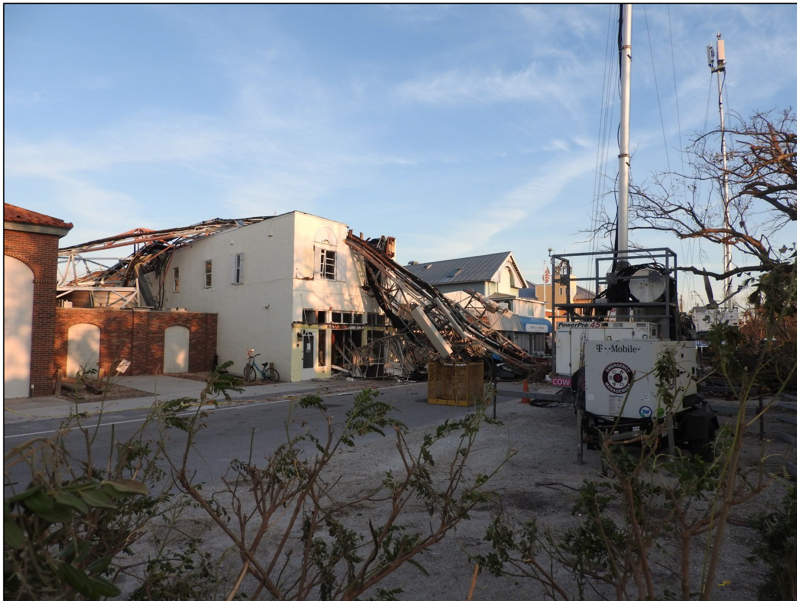
Figure 31. Collapse of an older cell tower onto the local bakery in Boca Grande from hurricane winds landward of R-14.
