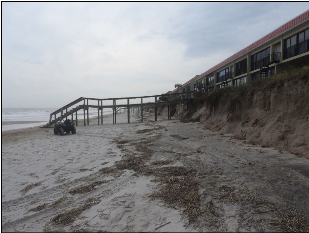
Figure 56. Major beach and dune erosion in Ponte Vedra (R-15).
