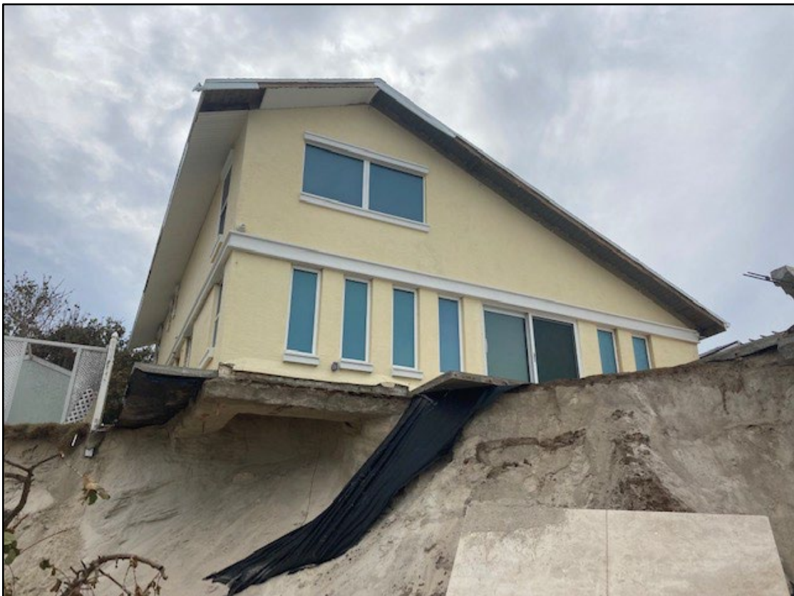
Figure 114. House in imminent danger of collapse, Wilbur-by-the-Sea (R125).
