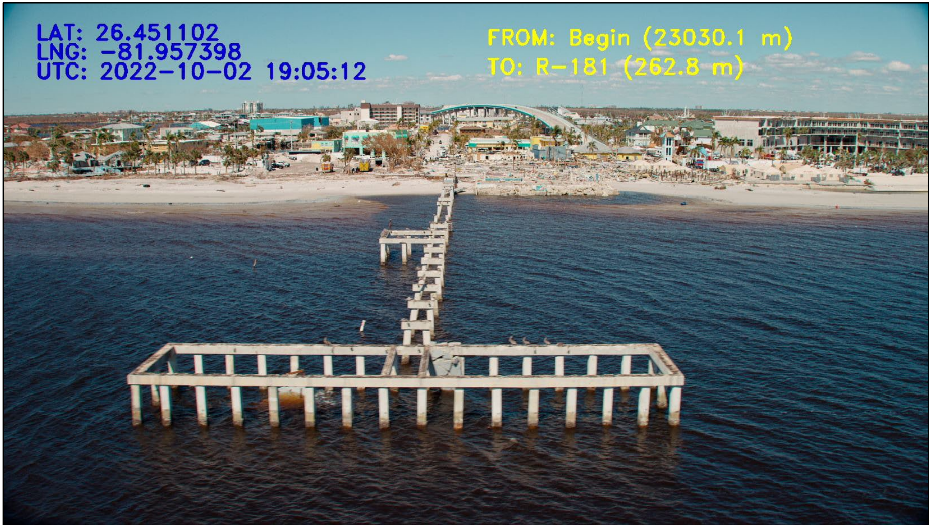
Figure 38. Ft. Myers Beach structures and pier with major damages, R-181 (Image source: Active Camera Systems and Camera Copters).
