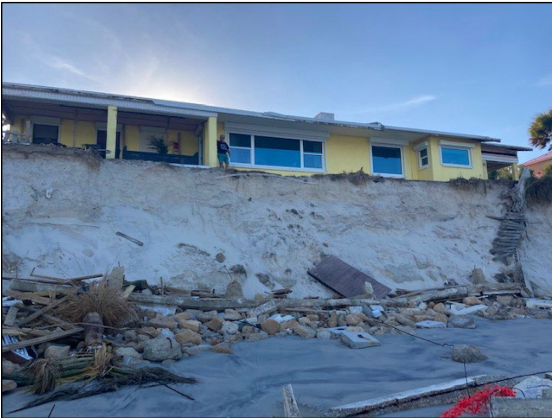
Figure 95. Wilbur-by-the-Sea dwelling threatened following seawall failure (R125).
