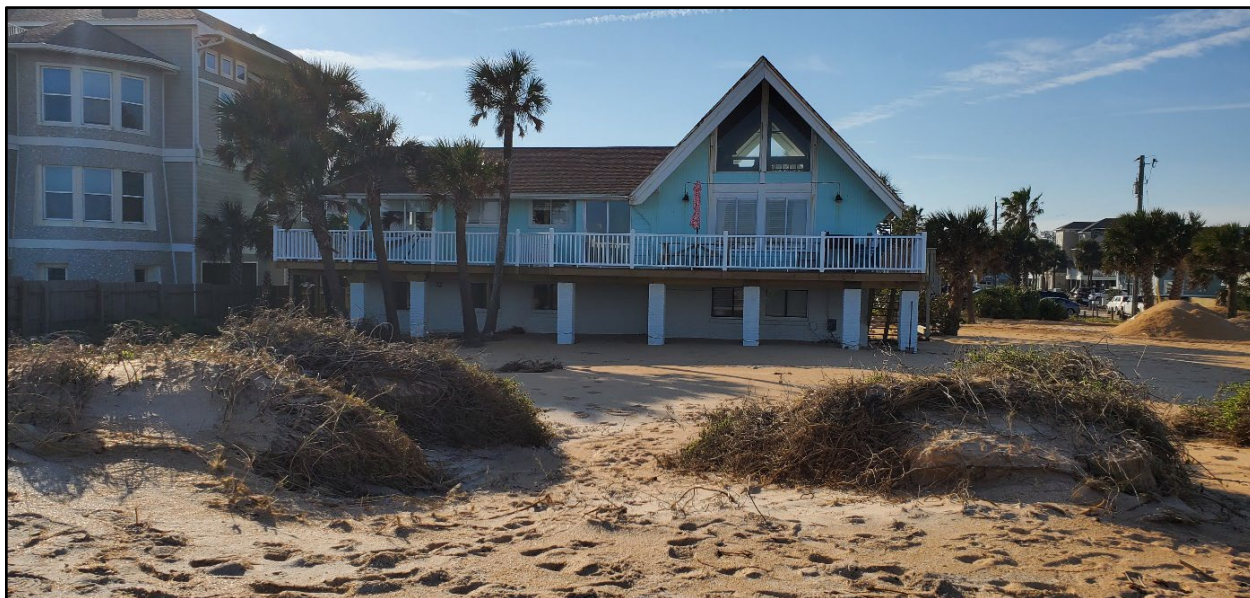
Figure 71. Home flooded and sanded south of Seascapes Drive (R-17).
