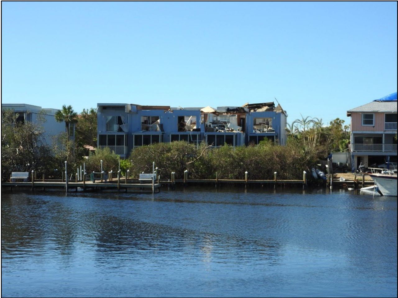
Figure 21. Condominiums destroyed in Englewood Beach (R-11).
