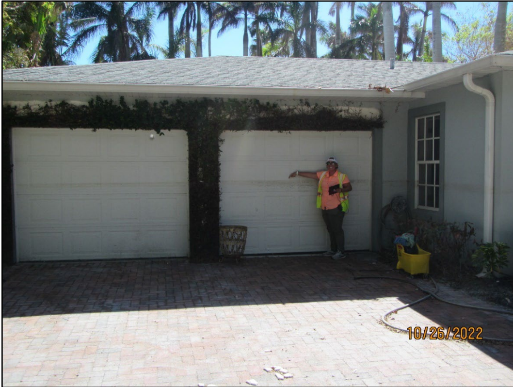
Figure 52. High water mark shown on a single-family dwelling, Naples (R-71).
