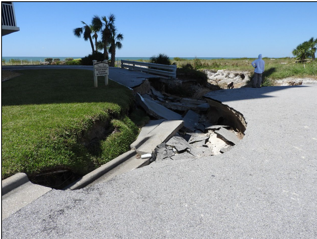
Figure 16. Storm water runoff gullies at Alhambra Road, Venice Beach (R-122).
