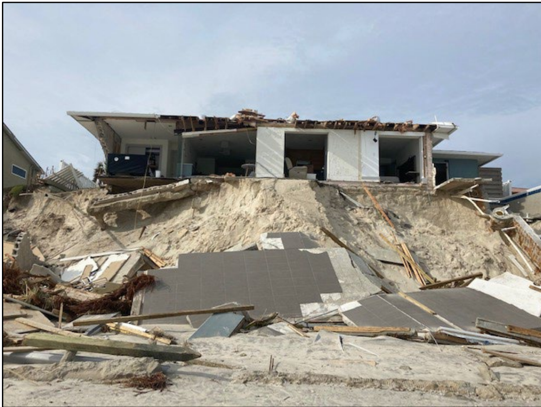
Figure 109. House destroyed, Wilbur-by-the-Sea (R125).
