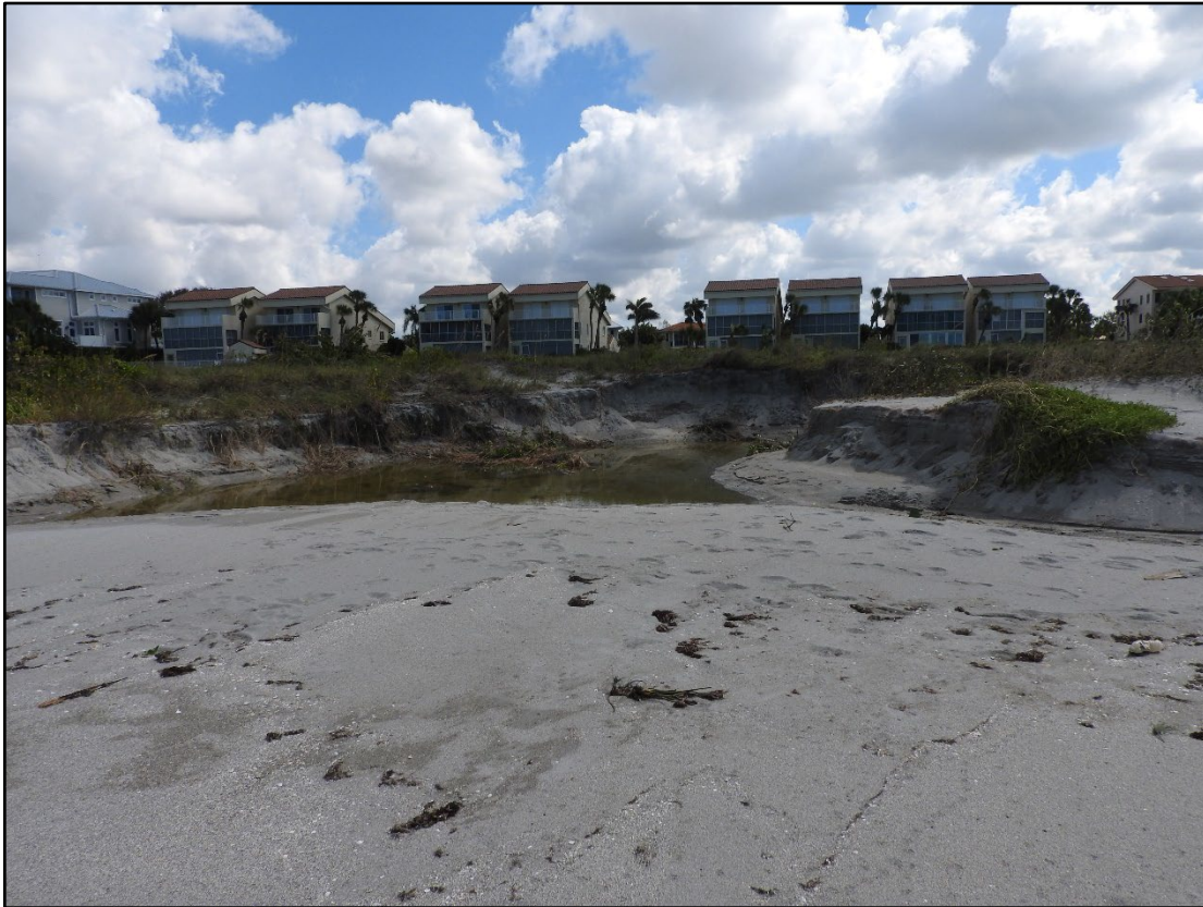
Figure 15. Storm water runoff gullies, Venice Beach (R-127).
