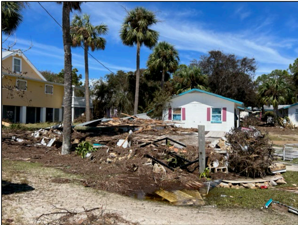
Figure 42. A motel building destroyed by the storm surge and waves, G Street, Cedar Key.
