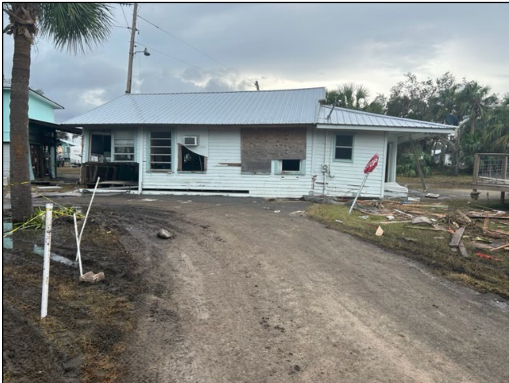
Figure 34. A dwelling floated onto a road intersection at Horseshoe Beach.
