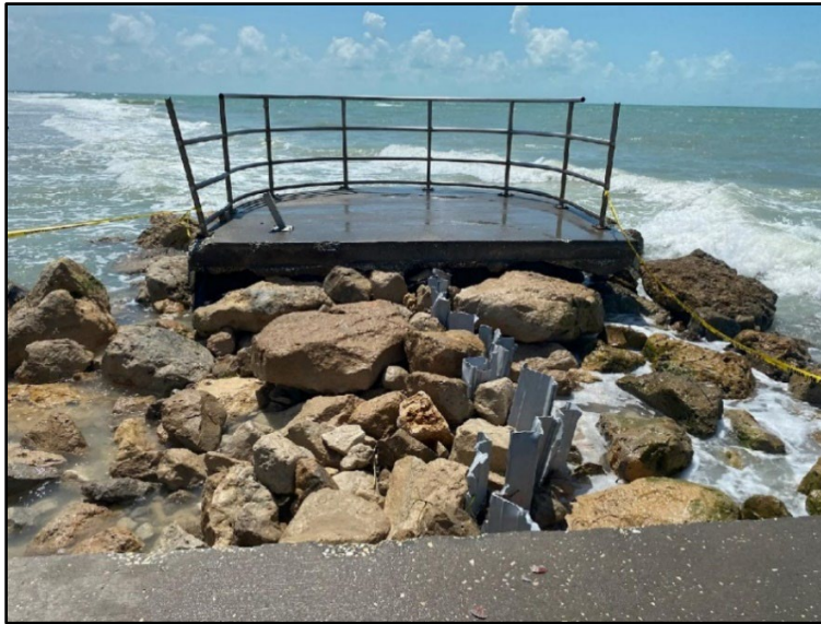
Figure 55. Major damage to John's Pass south jetty (photo courtesy of Zach Westfall with Pinellas County).
