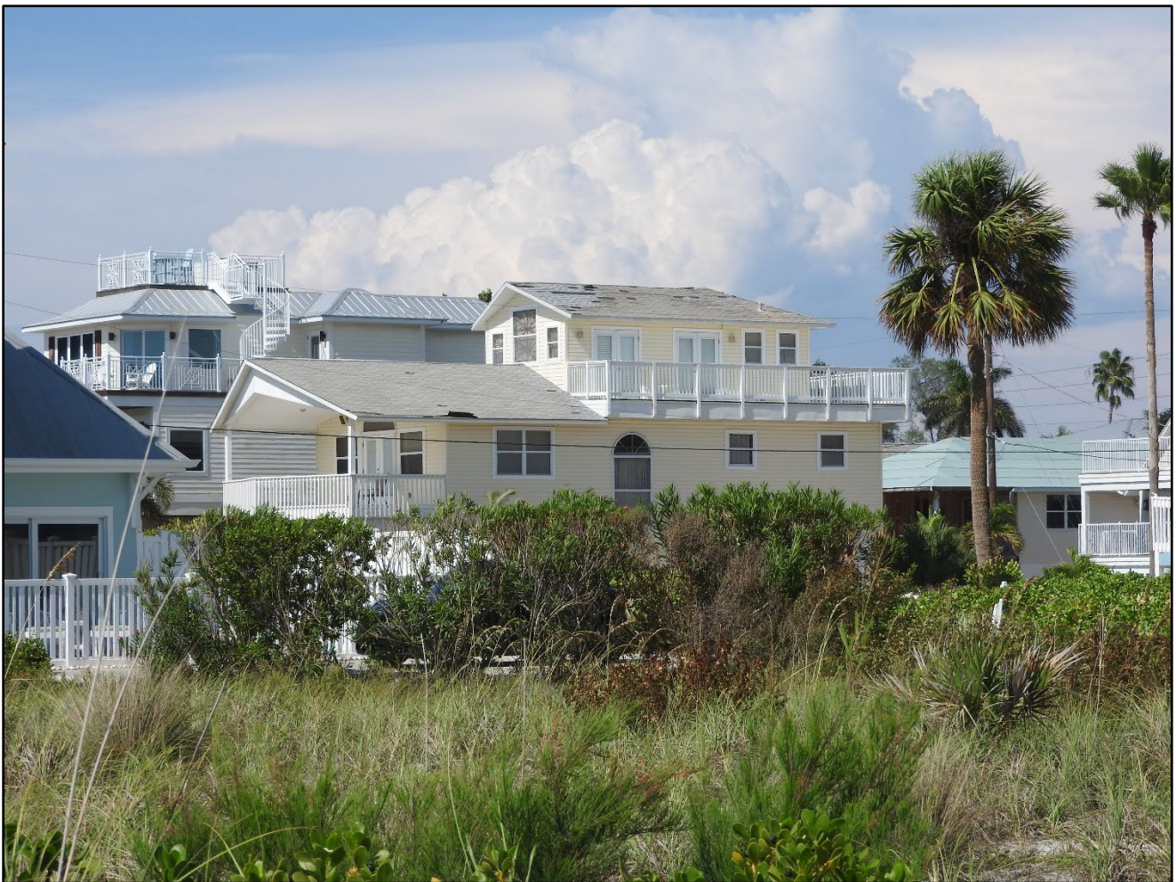
Figure 56. Roofing damage on Anna Maria Island, near R25.
