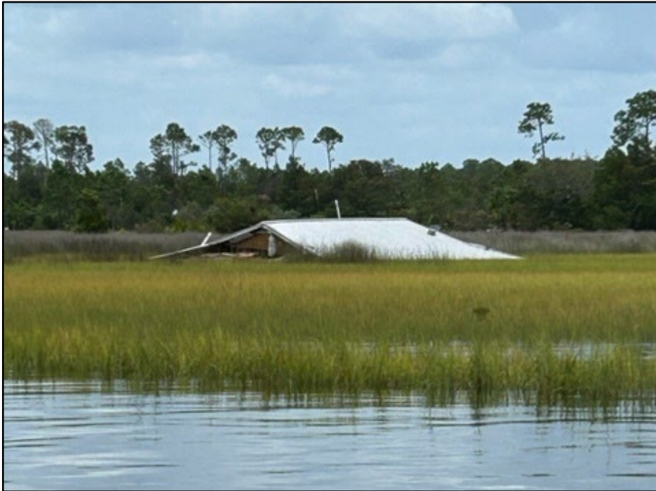
Figure 38. A roof carried into wetlands from dwelling below.
