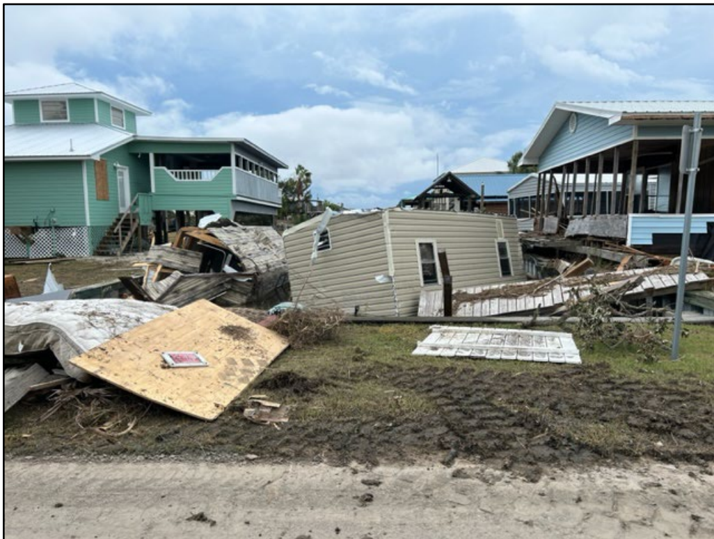
Figure 35. Buildings and other debris in a canal, Horseshoe Beach.
