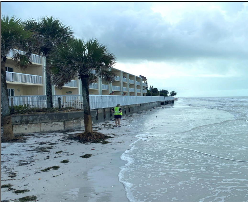
Figure 477. Post-Hurricane Idalia at the Fifty Gulfside Condominium in Indian Shores on Sand Key, R84 (photo courtesy of Zach Westfall of Pinellas County).
