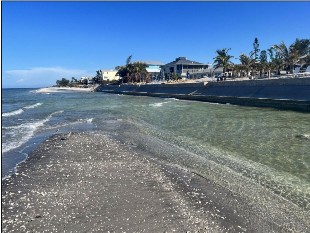
Figure 67. Beach and dune erosion on Manasota Key at R14.5 (photo courtesy of Vadim Alymov with Coastal Engineering Consultants, Inc.).
