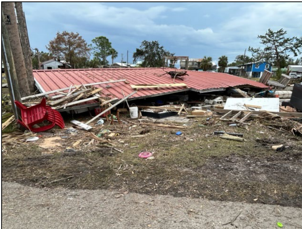
Figure 33. Dwelling destroyed in Horseshoe Beach.
