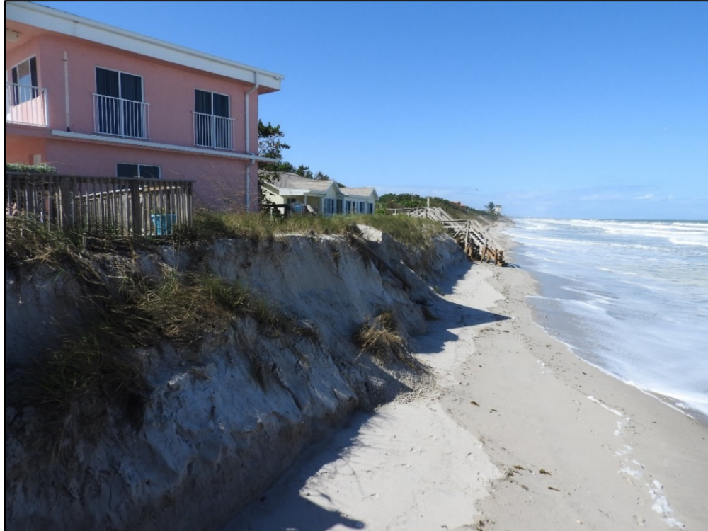
Figure 20a. Major beach and dune erosion threatening structures in south Brevard County (R151).
