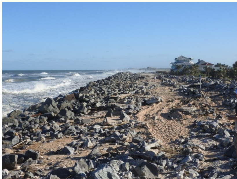
Figure 17g. Major damage to the federal rock revetment and total loss of Old AIA at Summer Haven, St. Johns County (R199).
