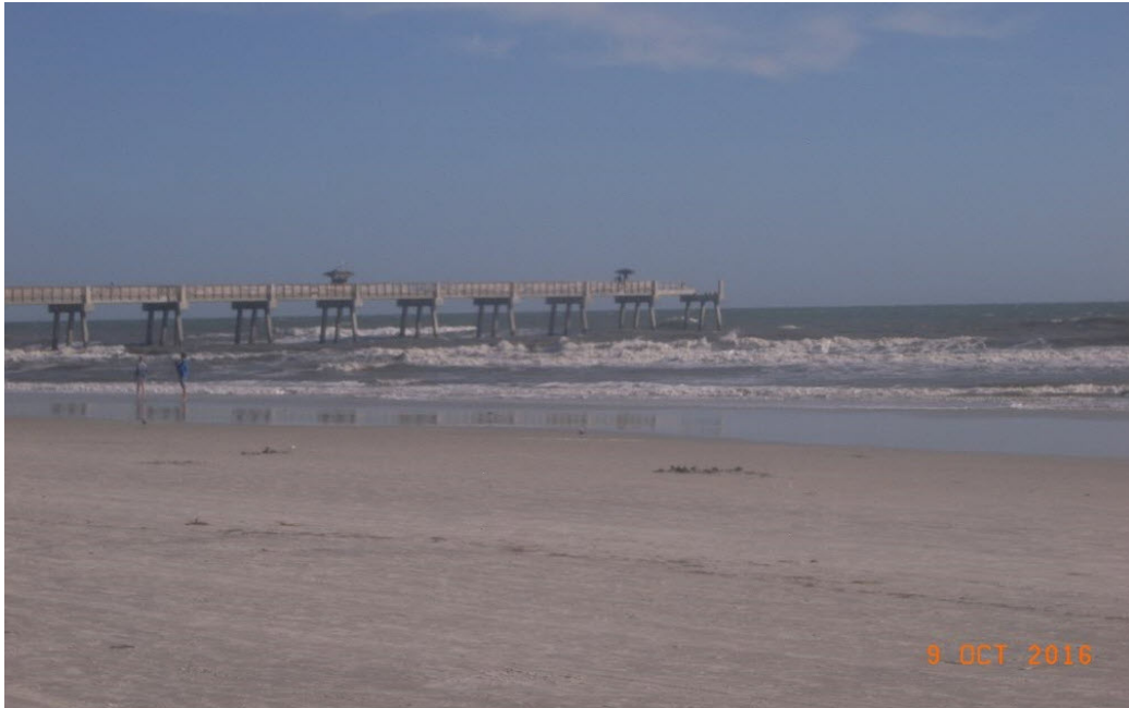
Figure 16a. Over 300 feet of the eastern end of the Jacksonville Beach Fishing Pier was destroyed, Duval County (R65).
