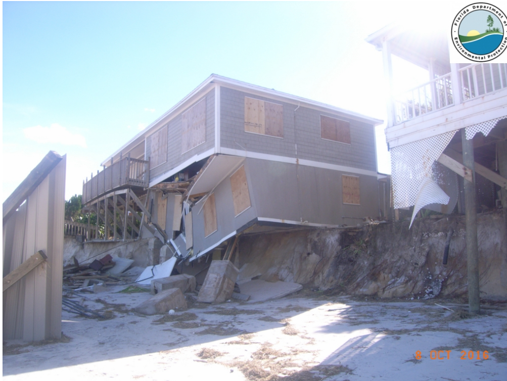
Figure 17c. Major dune erosion and major structural damage to a single-family dwelling in South Ponte Vedra, St. Johns County (R87).
