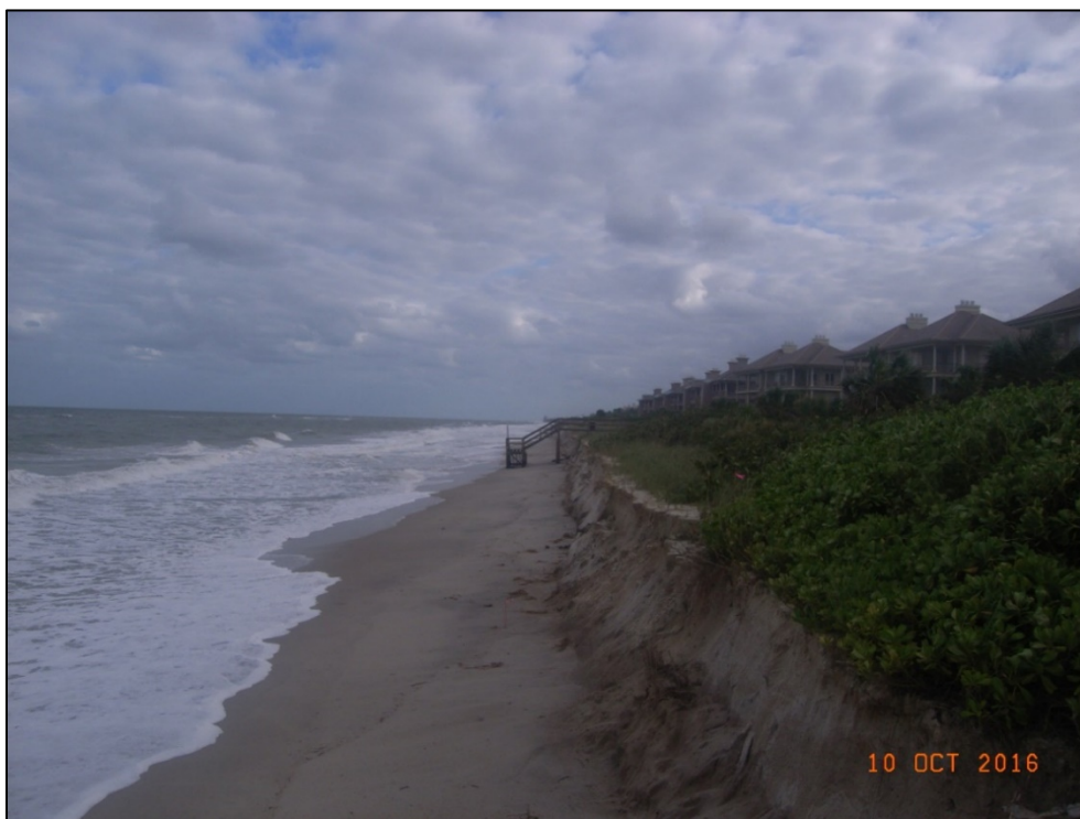
Figure 21b. Major beach and dune erosion with a 10-foot high vertical scarp in Indian River County (R34).
