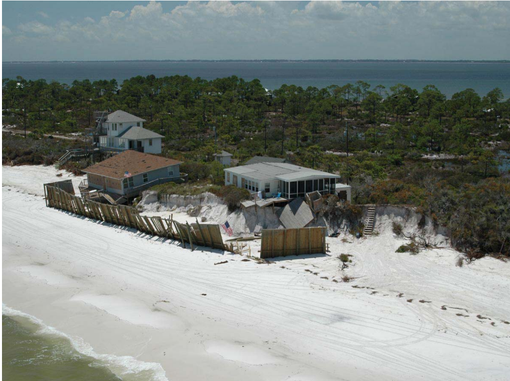
Photo 7. Wood bulkhead destroyed (R171)
