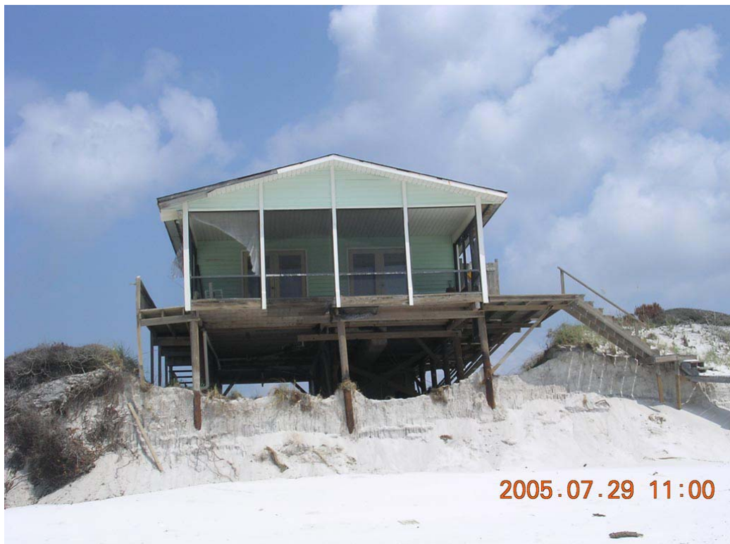
Photo 4. Imminently endangered pile-supported dwelling (R175)
