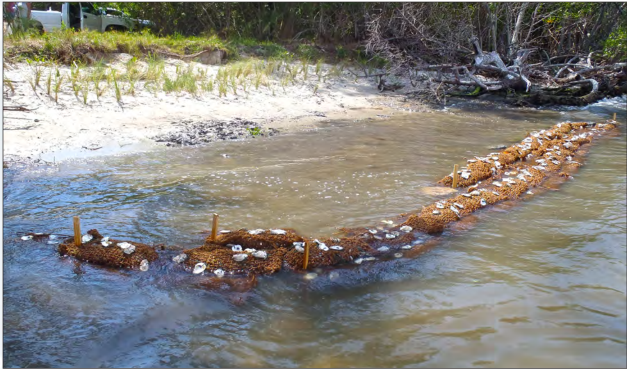
As part of the Shoreline Restoration Project, IRLAP staff conducts projects to stabilize eroding shorelines. Oyster reef restoration helps to attenuate wave action, provide habitat, and protect coastal plantings.
