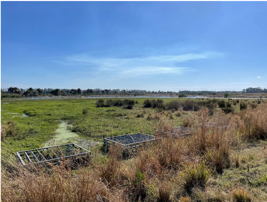
NRCS Wetland Reserve Easement and associated control structures
