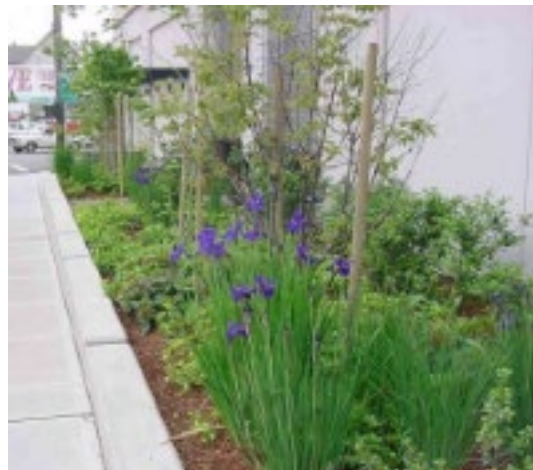
Figure 5-13. Sidewalk infiltration planter box.
