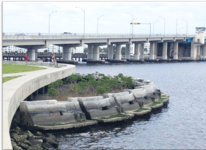
Figure 2-15. Living shoreline mangrove planter in Lake Worth Beach. (Photo: Michael Singer Studio)
