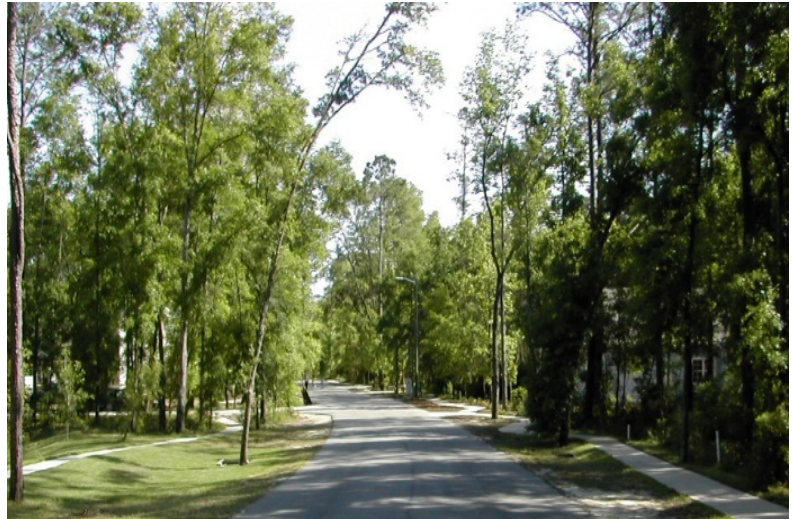
Figure 4-3. Roadside swales replace curbs and gutters along a residential street. (Photo: UF PREC)
