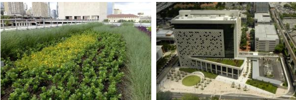
Figure 5-6. Views of the green roof at Miami-Dade Children's Courthouse.
