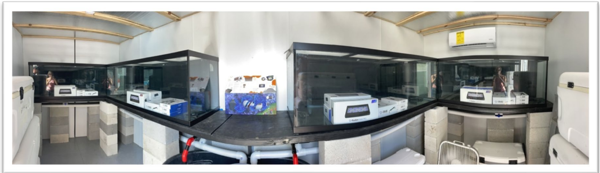
Figure 4 TRI shipping container installed.
