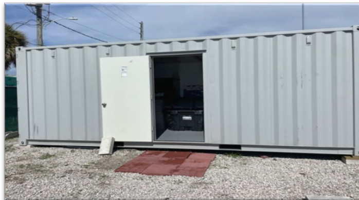
Figure 3 TRI shipping container installation.
