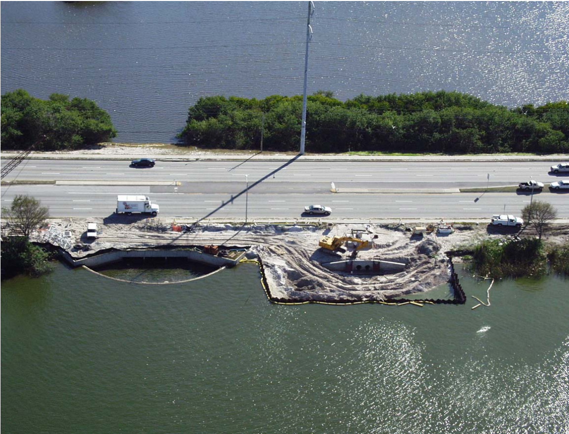
Photo 3-5. Photograph of outfall structure under construction.
