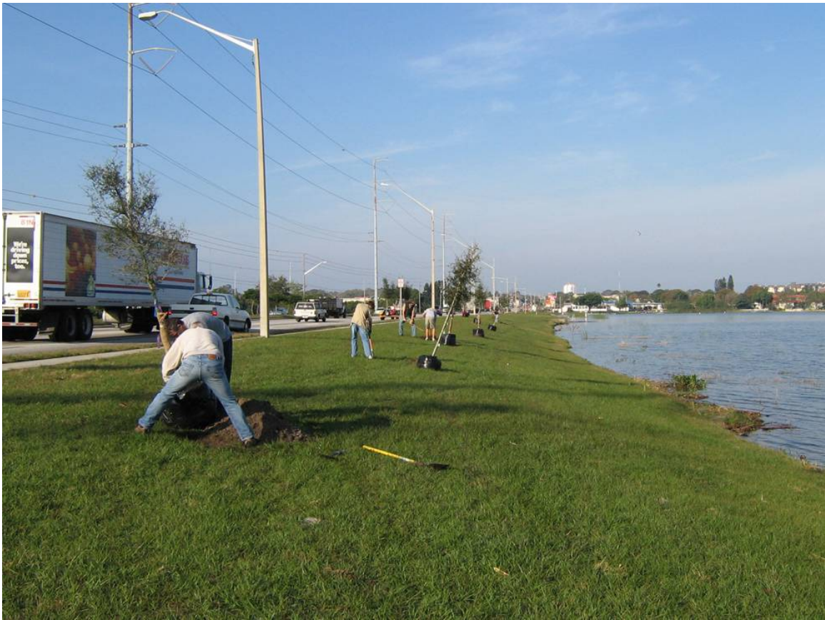
Photo 3-7. Installation of 30 live oaks along Park Blvd by Eagle Scouts.
