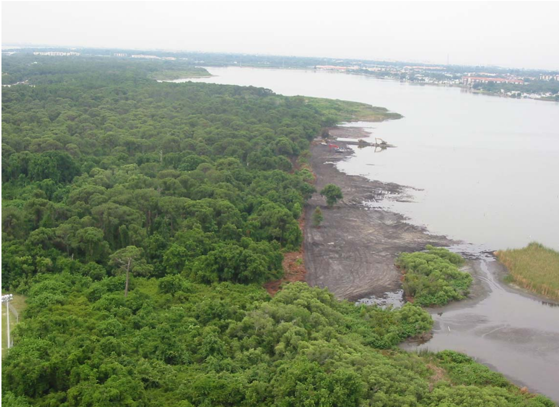
Photo 3-1. Organic sediment removal for shoreline restoration in Lake Seminole.
