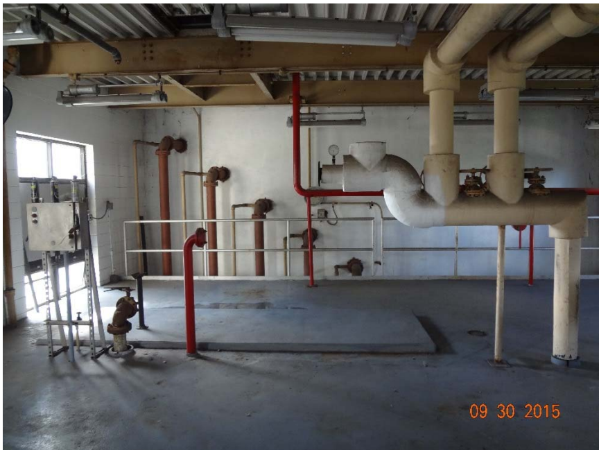
Figure NWWRF-10. Anaerobic Digester Building Third Floor Northwest WRF
