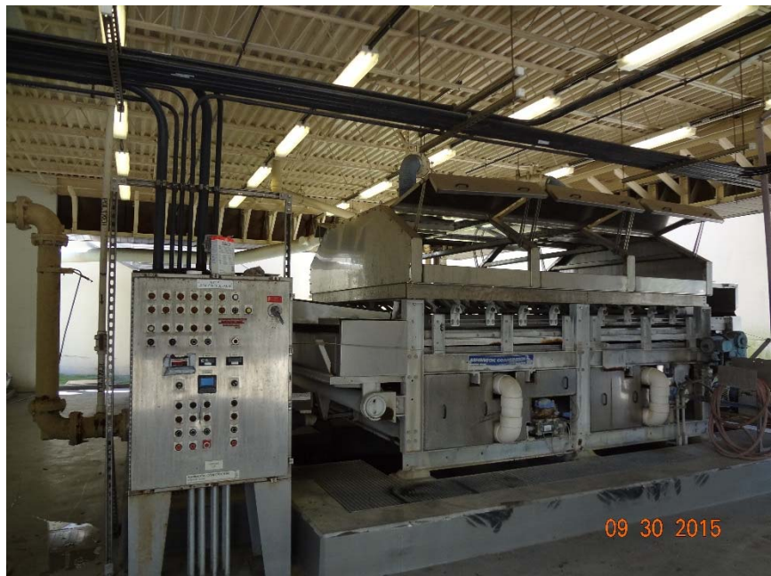
Figure SWWRF-2. Gravity Belt Thickener Southwest WRF
