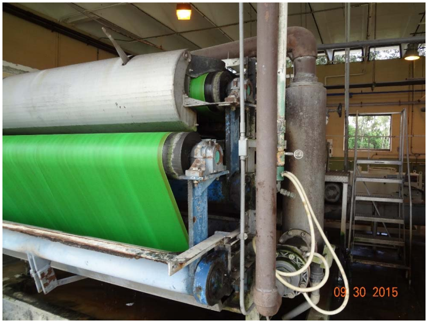
Figure SWWRF-7. Belt Filter Press Southwest WRF
